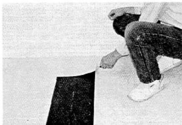
Removal of tile over subfloor joint.
