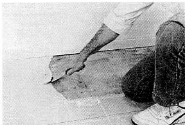
Scrape from remaining floor covering.
