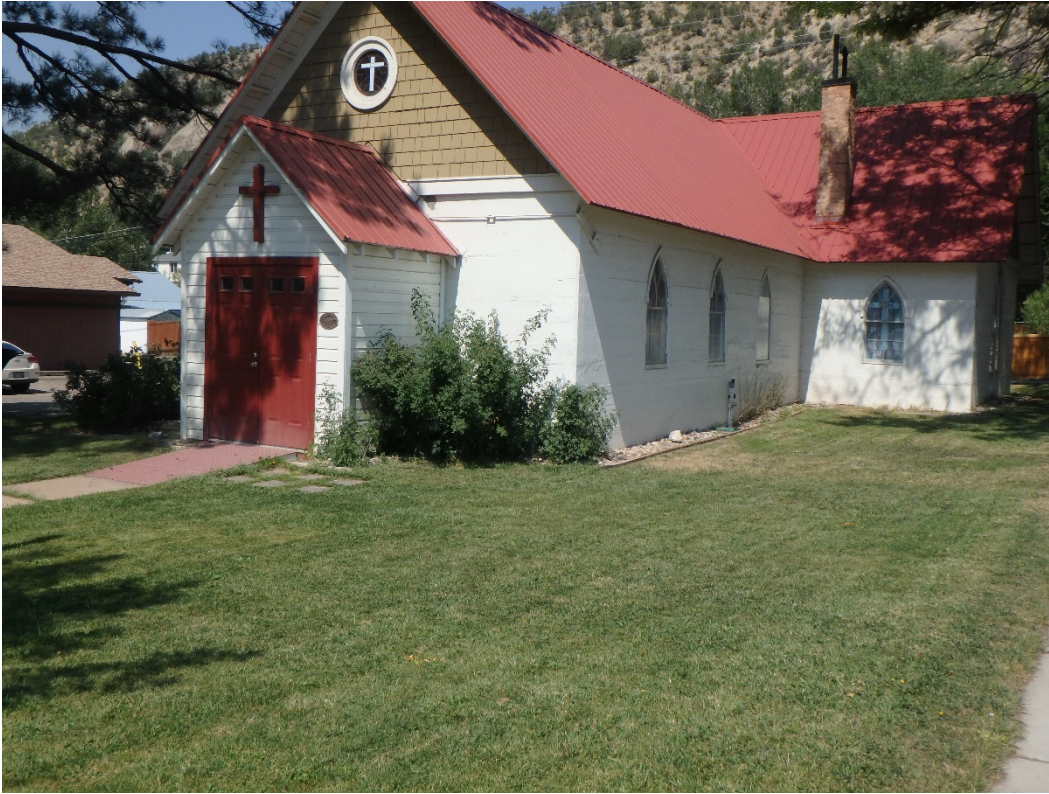
Photo Number: 5GF.2368_1 Description: Looking at the primary (south) and east elevations of the building. Note the historic brick masonry chimney; exposed rafter tails under the eaves; and the gothic arch window units. Date: 9/6/2022 View: Northwest
