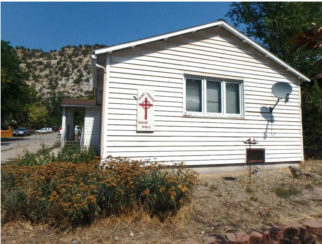
Photo Number: 5GF.5921_2 Description: Looking at the south elevation of the building. Date: 9/6/2022 View: North
