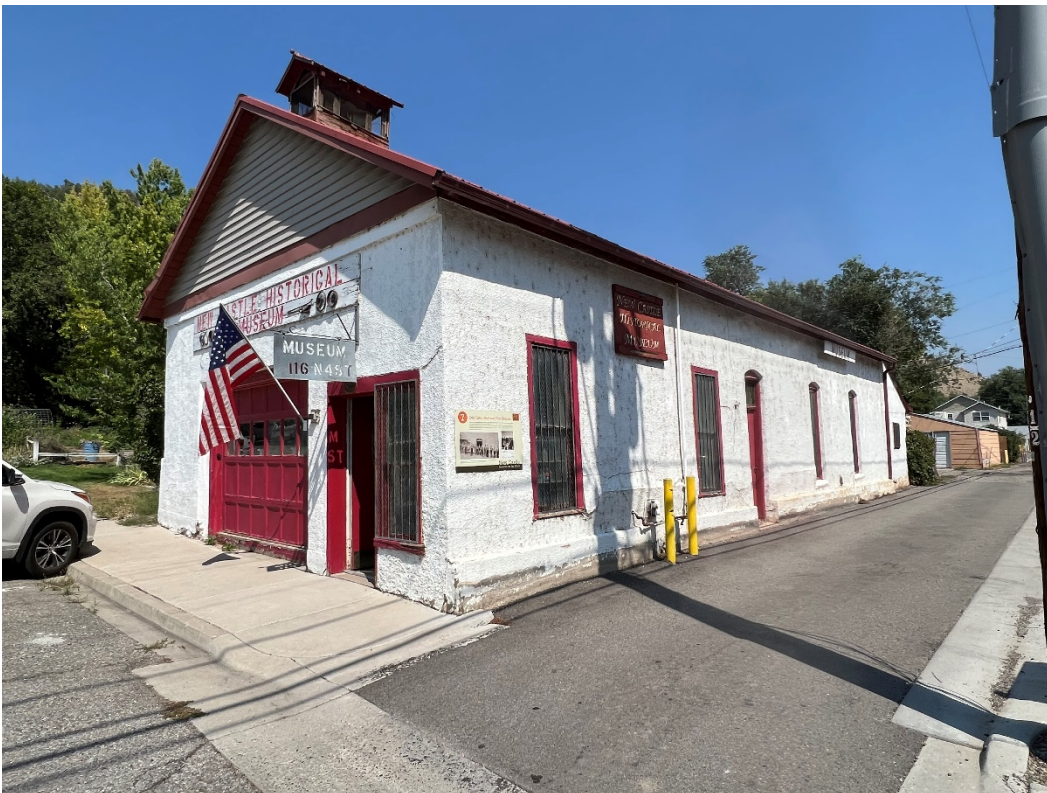
Photo Number: 5GF.1665_2 Description: Looking at the primary (west) and south elevations of the building. Date: 9/6/2022 View: Northeast
