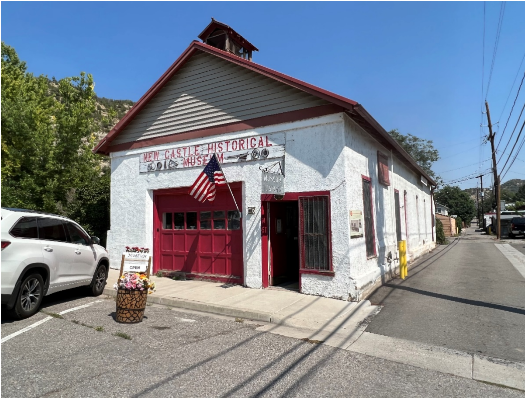
Photo Number: 5GF.1665_1 Description: Looking at the primary (west) and south elevations of the building. Date: 9/6/2022 View: Northeast
