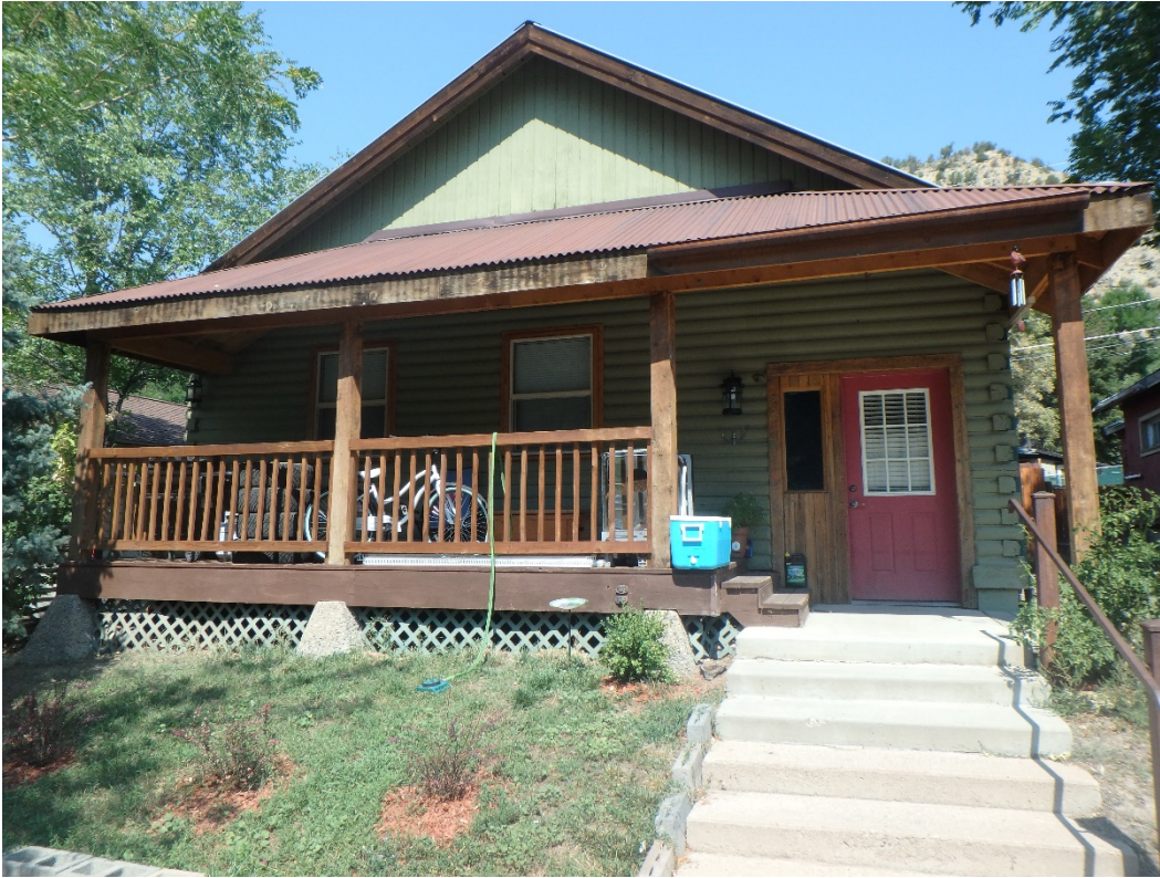
Photo Number: 5GF.5922_1 Description: Looking at the primary (south) elevation of the building. Date: 9/6/2022 View: North
