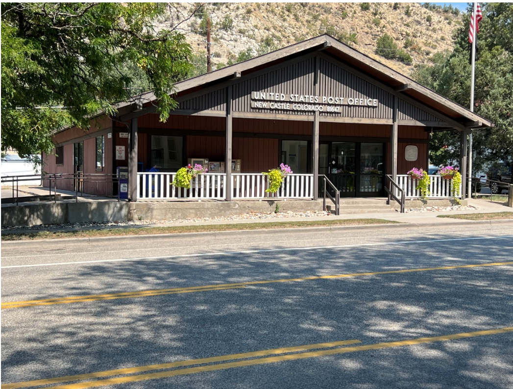
Photo Number: 5GF.5890_2 Description: Looking at the west and primary (south) elevations of the building. Date: 9/6/2022 View: Northeast
