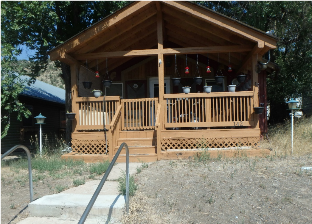
Photo Number: 5GF.5923_1 Description: Looking at the primary (south) elevation of the building. Note the decorative arrangement of the overhang support posts and the woodwork along the facade. Date: 9/6/2022 View: North
