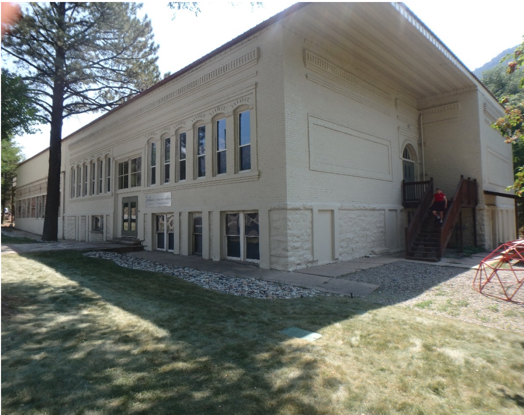
Photo Number: 5GF.2369_1 Description: Looking at the primary (north) and west elevations of the building. Note the several ornate brickwork features along the facade. Date: 9/6/022 View: Southeast
