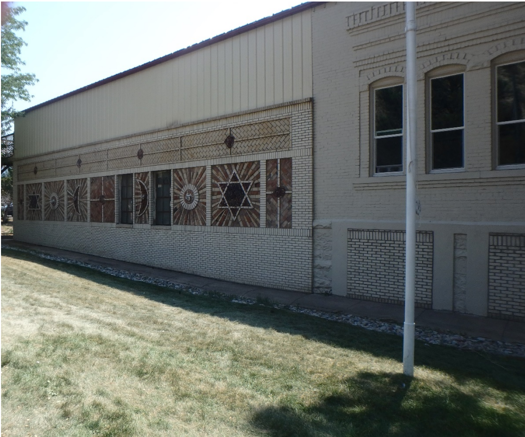
Photo Number: 5GF.2369_3 Description: Looking at the 1939 adobe brick addition to the original 1913 building. Date: 9/6/2022 View: Southeast
