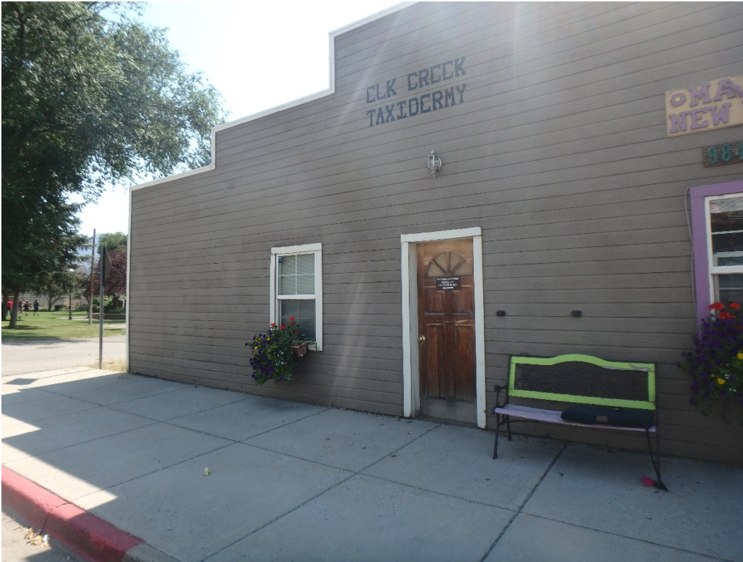
Photo Number: 5GF.5919_1 Description: Looking at the primary (north) elevation of the building. Note the false front that features a stepped parapet design. Date: 9/6/2022 View: Southeast
