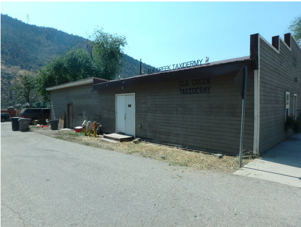
Photo Number: 5GF.5919_2 Description: Looking at the east and primary (north) elevations of the building. Date: 9/6/2022 View: Southwest
