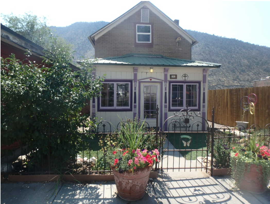
Photo Number: 5GF.2370_1 Description: Looking at the primary (north) elevation of the building. Note the 1976 enclosed porch addition to the façade. Date: 9/6/2022 View: South
