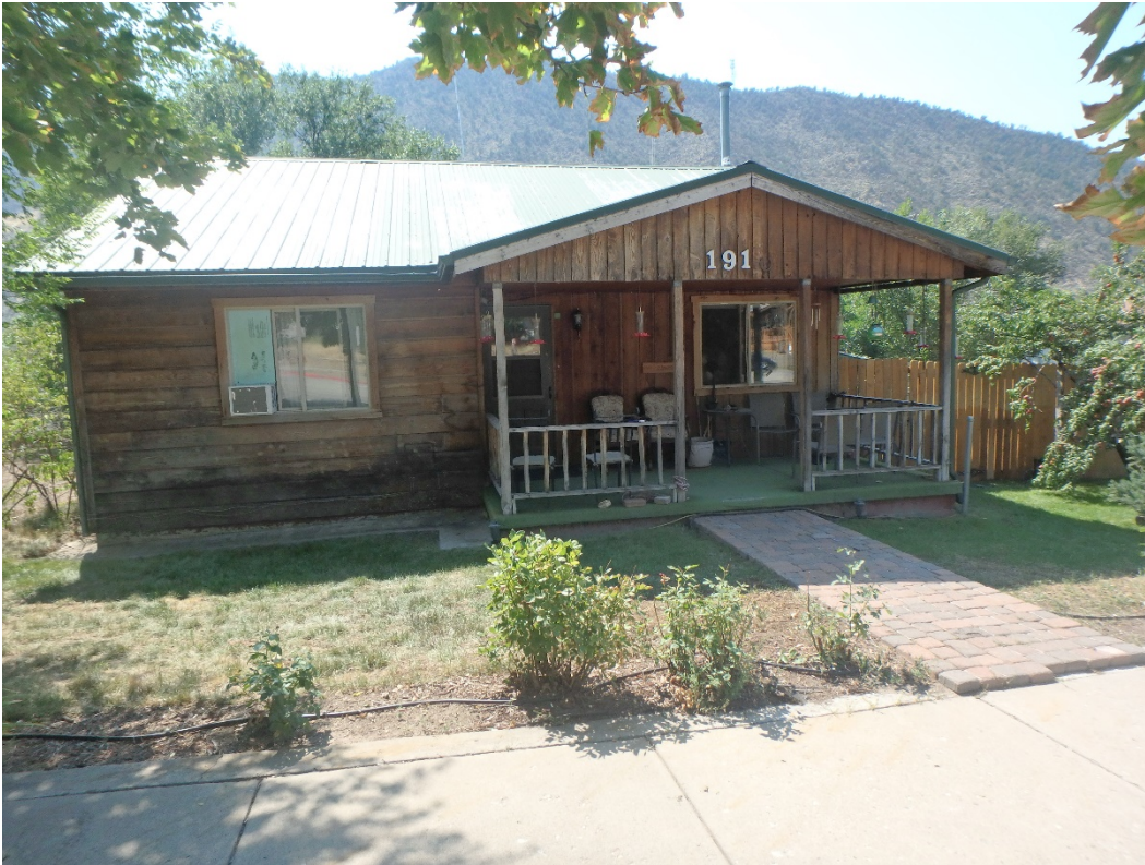
Photo Number: 5GF.5925_1 Description: Looking at the primary (north) elevation of the building. Date: 9/6/2022 View: South
