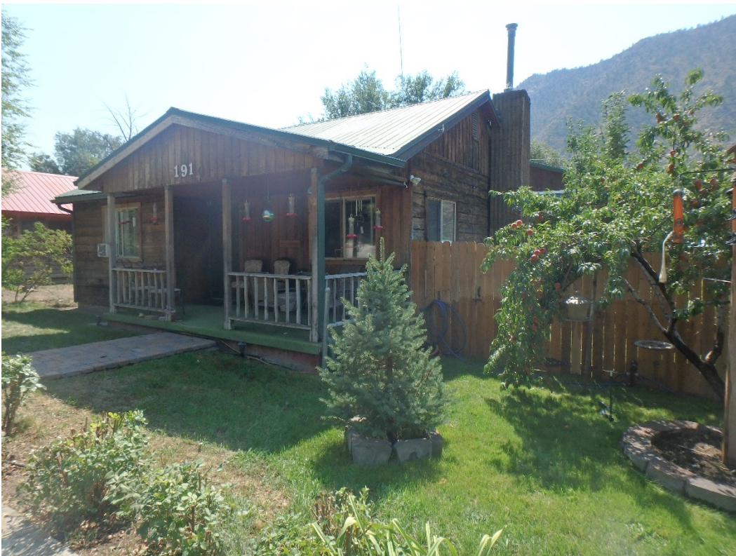
Photo Number: 5GF.5925_2 Description: Looking at the primary (north) and west elevations of the residence. Date: 9/6/2022 View: Southeast
