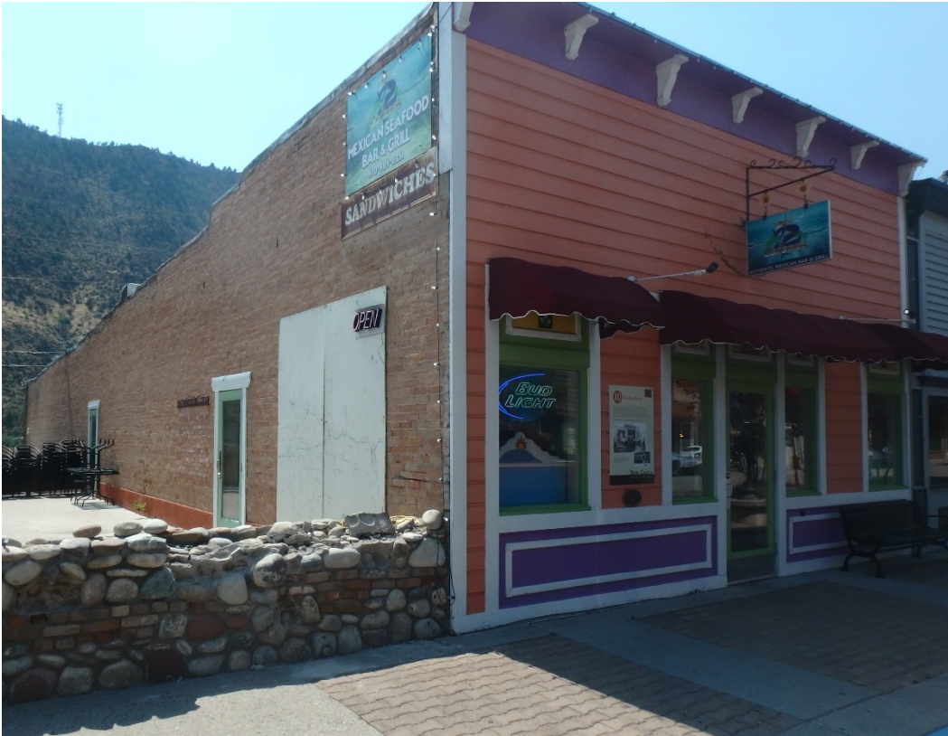
Photo Number: 5GF.2371_1 Description: Looking at the east and primary (north) elevations of the building. Date: 9/6/2022 View: Southwest
