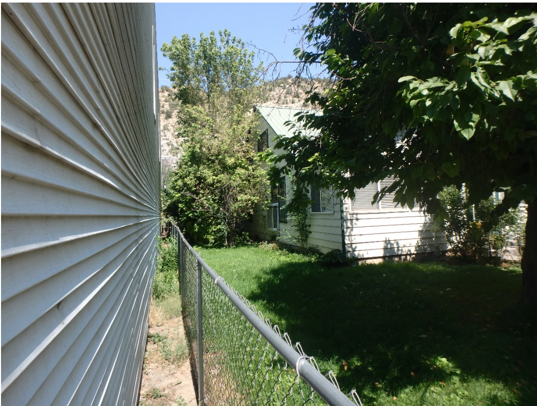
Photo Number: 5GF.5918_2 Description: Looking at the west and primary (south) elevation of the building. Note that the wall to the left is not a part of the residence. Date: 9/6/2022 View: Northeast
