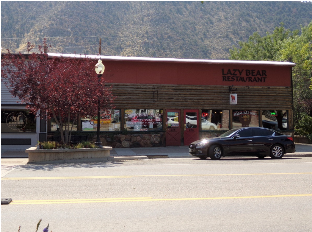
Photo Number: 5GF.2374_1 Description: Looking at the primary (north) elevation of the building. Date: 9/6/2022 View: South
