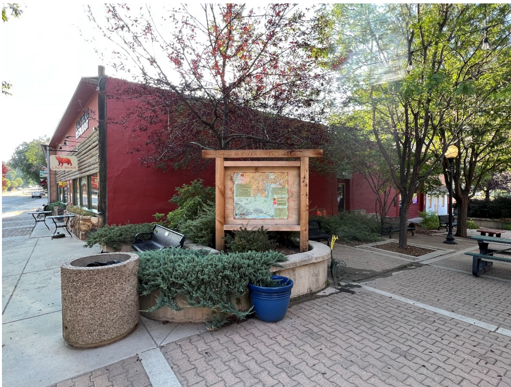
Photo Number: 5GF.2374_2 Description: Looking at the primary (north) and west elevations of the building. Date: 9/6/2022 View: Southeast
