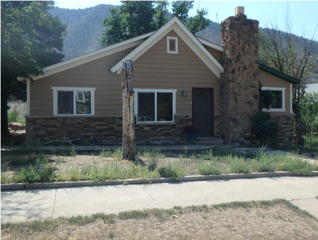
Photo Number: 5GF.5928_1 Description: Looking at the primary (north) elevation of the residence. Date: 9/6/2022 View: South
