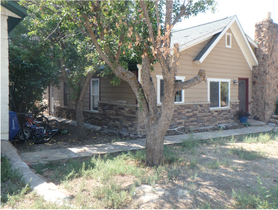
Photo Number: 5GF.5928_3 Description: Looking at the west and primary (north) elevations of the building. Date: 9/6/2022 View: Southwest
