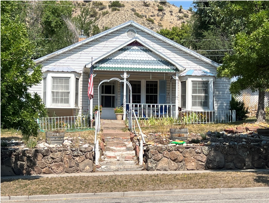
Photo Number: 5GF.5929_1 Description: Looking at the primary (south) elevation of the primary building. Note the decorative wood spindlework and brackets under the gable ceiling of the porch overhang. Date: 9/6/2022 View: North
