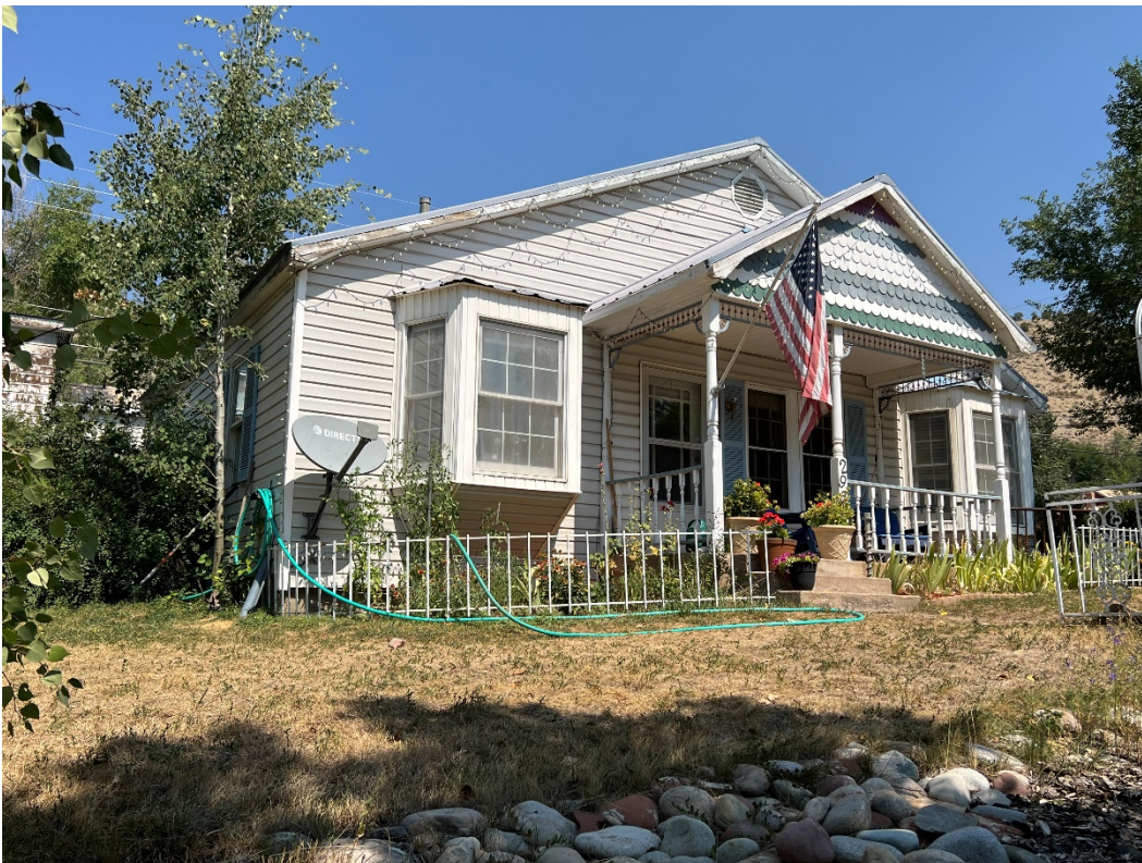
Photo Number: 5GF.5929_2 Description: Looking at the west and primary (south) elevations of the primary residence. Date: 9/6/2022 View: Northeast
