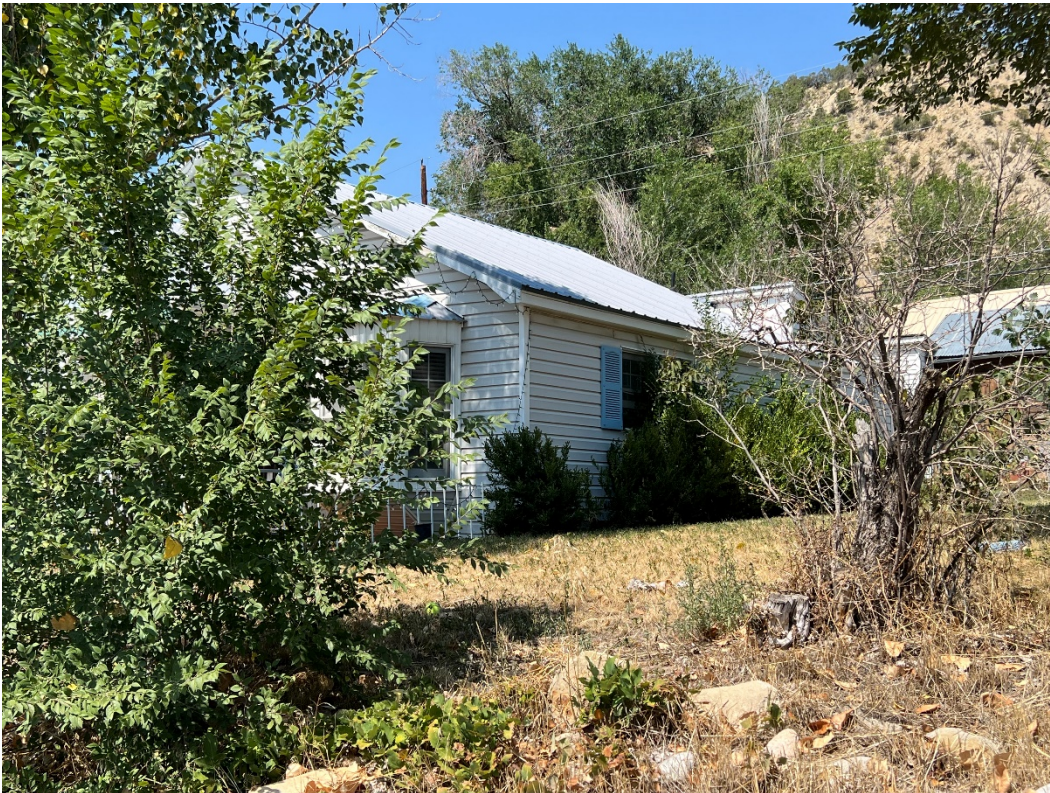
Photo Number: 5GF.5929_4 Description: Looking at the east elevation of the primary building. Date: 9/6/2022 View: Northwest
