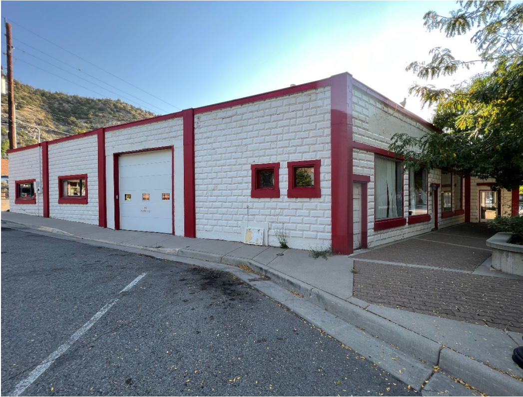
Photo Number: 5GF.2373_3 Description: Looking at the west and primary (south) elevation of the building. Date: 9/6/2022 View: Northeast
