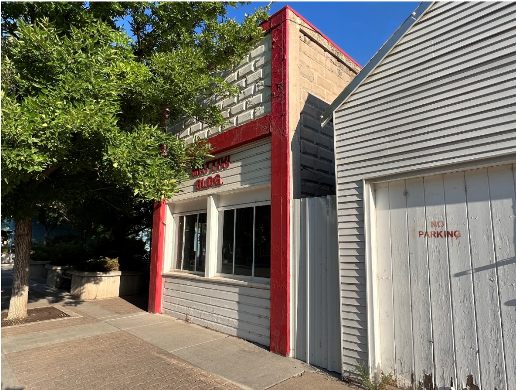
Photo Number: 5GF.2373_4 Description: Looking at the far-right side of the primary (south) and a portion of the east elevations. Note the former garage door opening that was covered by the mid to late Twentieth Century. Date: 9/6/2022 View: Northwest
