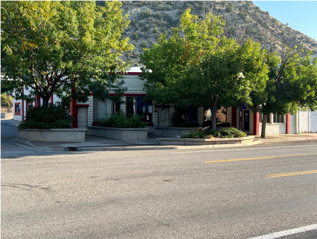
Photo Number: 5GF.2373_1 Description: Looking at the west and primary (south) elevations of the building. Note that a majority of the primary (south) elevation is obscured by mature deciduous trees. Date: 9/6/2022 View: Northeast
