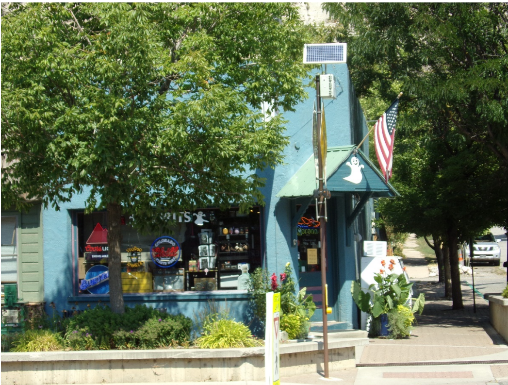
Photo Number: 5GF.2375_2 Description: Looking at the primary (south) elevation of the building. Date: 9/6/2022 View: North
