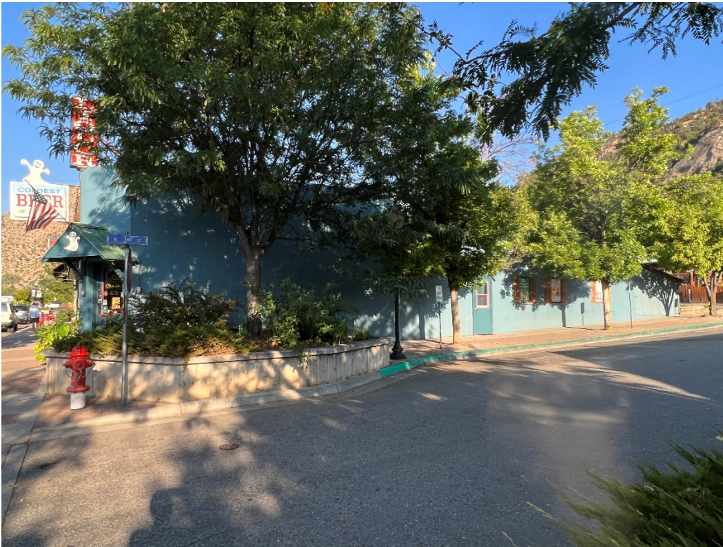
Photo Number: 5GF.2375_3 Description: Looking at the east elevation of the building. Note that a majority of the elevation is observed by landscaping features added between 1996 and 2005. Date: 9/6/2022 View: Northwest
