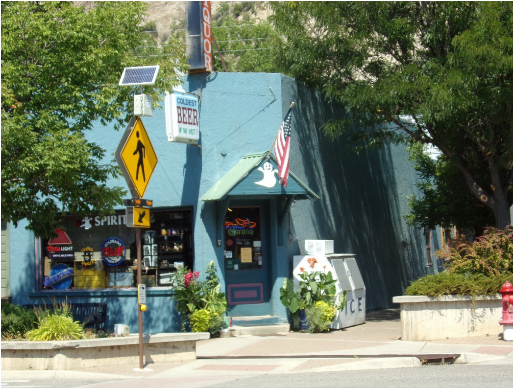
Photo Number: 5GF.2375_1 Description: Looking at the primary (south) and east elevations of the building. Date: 9/6/2022 View: Northwest
