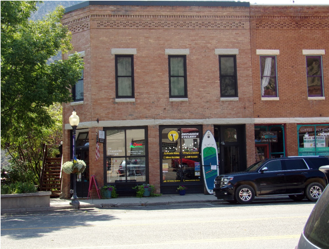
Photo Number: 5GF.2376_1 Description: Looking at the primary (north) elevation of the building. Note the decorative brickwork underneath the cornice. Date: 9/6/2022 View: South
