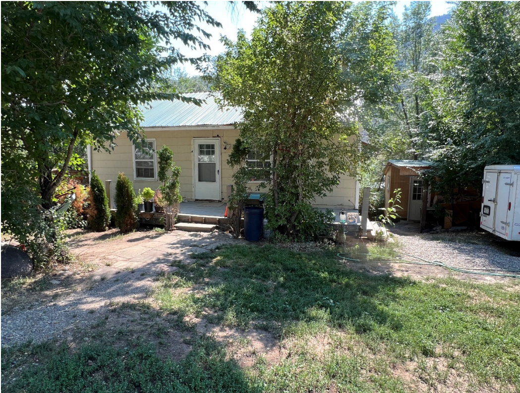
Photo Number: 5GF.5930_1 Description: Looking at the primary (north) elevation of the building. Date: 9/6/2022 View: South
