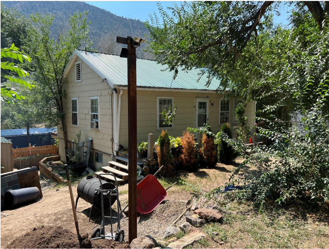
Photo Number: 5GF.5930_3 Description: Looking at the west and primary (north) elevations of the building. Date: 9/6/2022 View: Southwest
