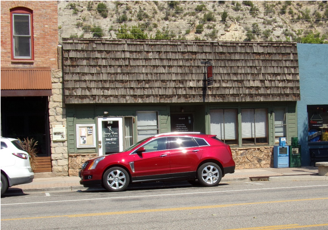
Photo Number: 5GF.2377_1 Description: Looking at the primary (south) elevation of the building. Date: 9/6/2022 View: North
