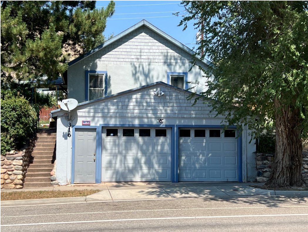
Photo Number: 5GF.5931_1 Description: Looking at the south elevation of the building. Date: 9/6/2022 View: North
