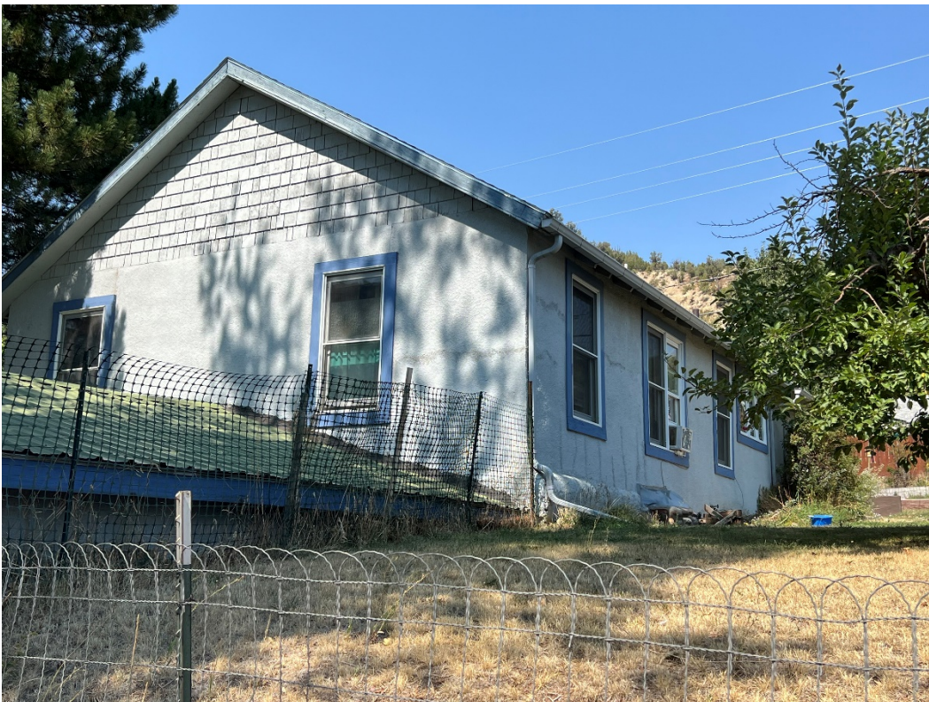
Photo Number: 5GF.5931_4 Description: Close up of the south and east elevations of the residence. Note the exposed rafter tails under the eaves that are partially obscured by the fascia board. Date: 9/6/2022 View: Northwest
