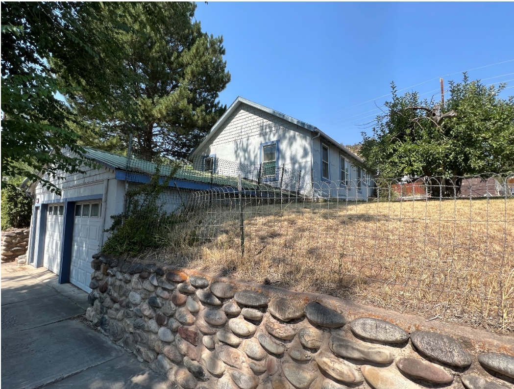
Photo Number: 5GF.5931_3 Description: Looking at the south and east elevations of the residence. Date: 9/6/2022 View: Northwest
