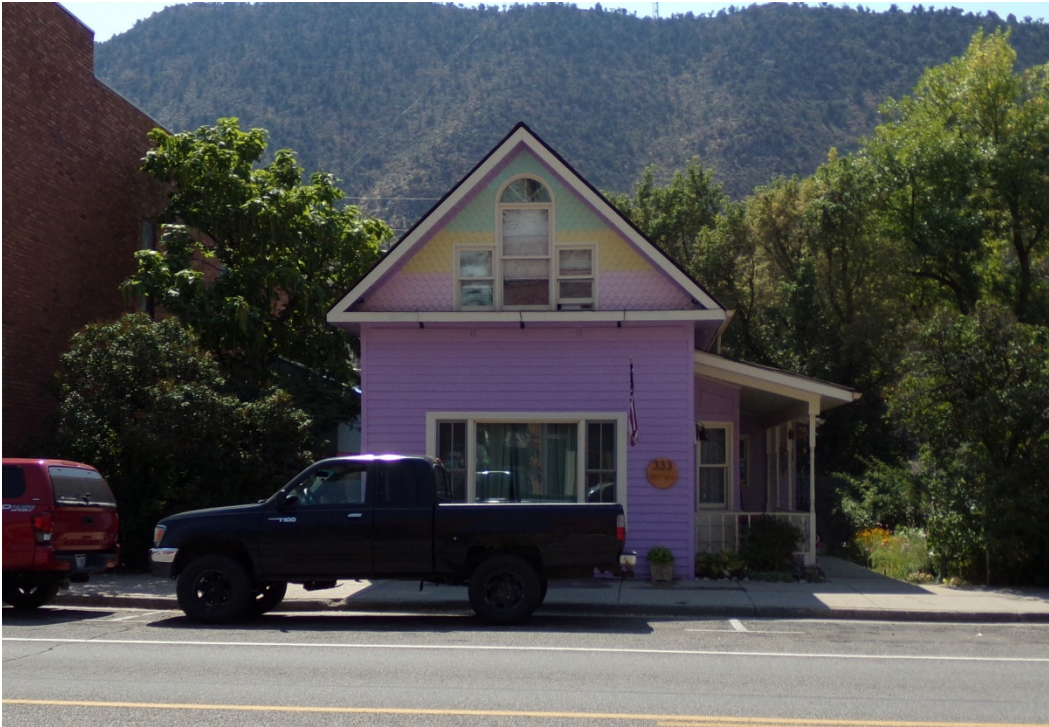
Photo Number: 5GF.5914_1 Description: Looking at the north elevation of the building. Date: 9/6/2022 View: South
