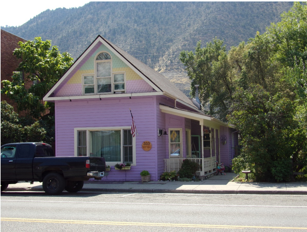
Photo Number: 5GF.5914_2 Description: Looking at the north and primary (west) elevations of the building. Date: 9/6/2022 View: Southeast
