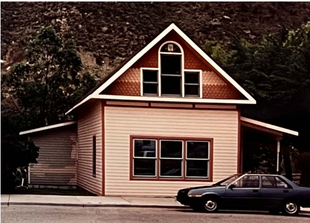
Reference Photo 1 Description: Looking at the west and north elevations of the residence. Date: Unknown Source: New Castle Museum Collection
