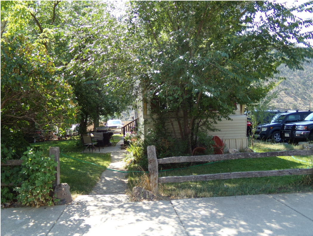
Photo Number: 5GF.5913_1 Description: Looking at the north elevation of the building. Date: 9/6/2022 View: South
