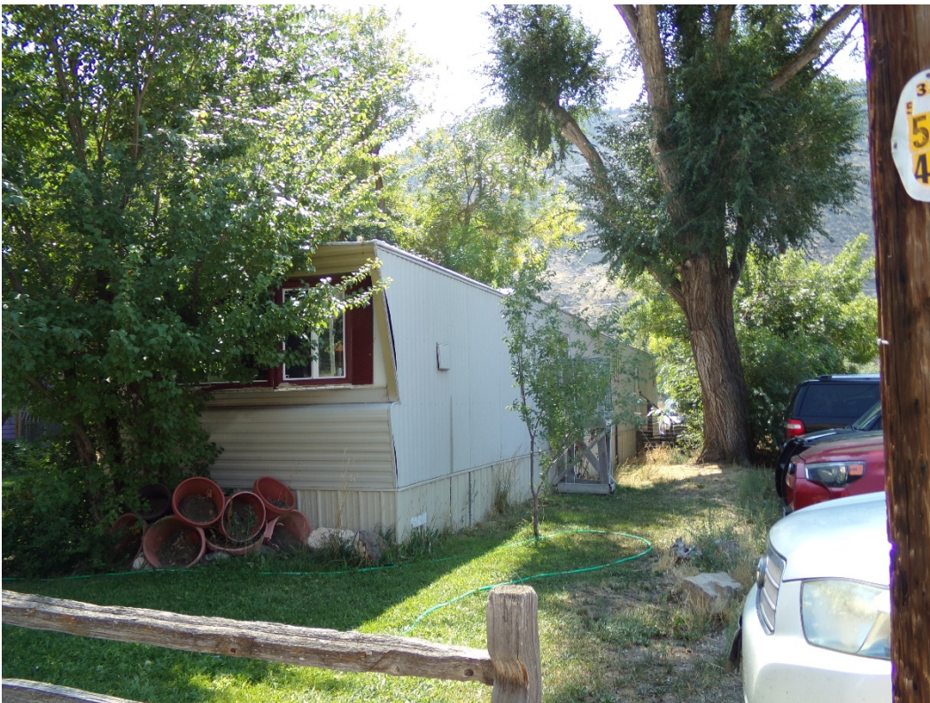
Photo Number: 5GF.5913_2 Description: Looking at the north and east elevations of the building. Date: 9/6/2022 View: Southeast
