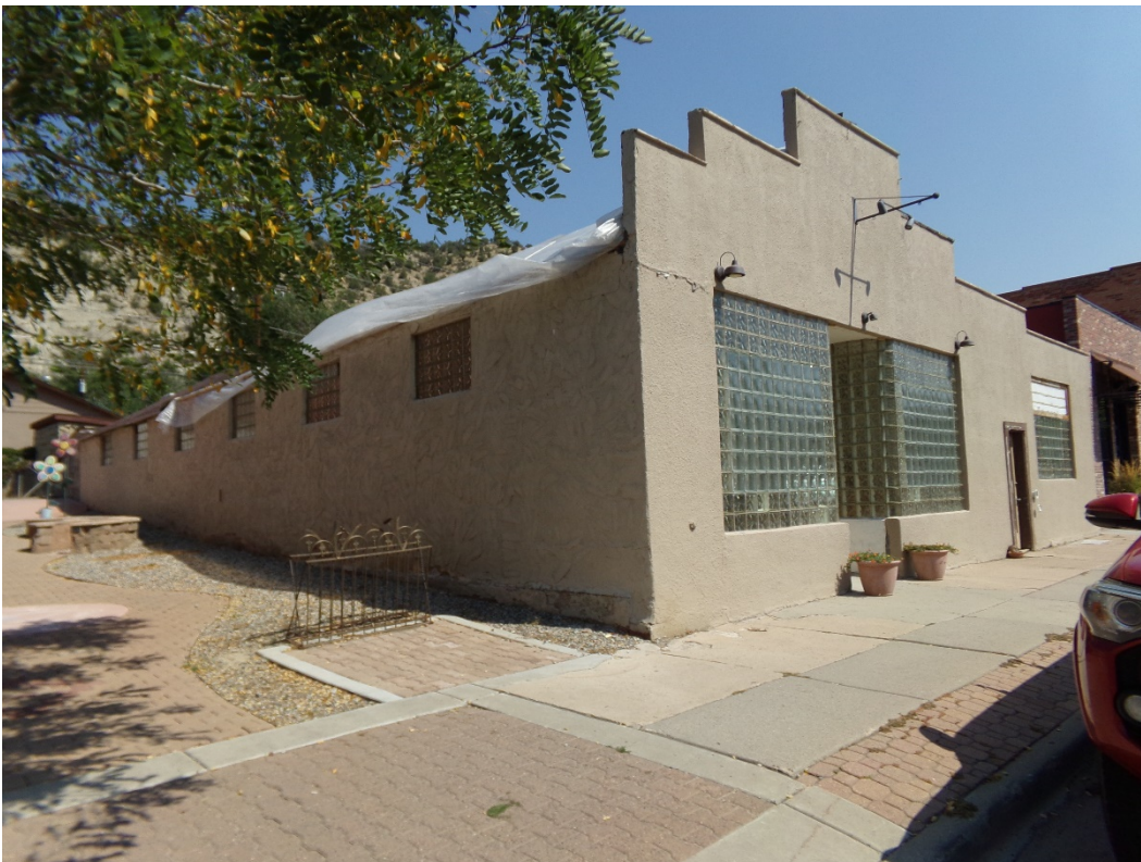
Photo Number: 5GF.5912_2 Description: Looking at the west and primary (south) elevations of the building. Date: 9/6/2022 View: Northeast
