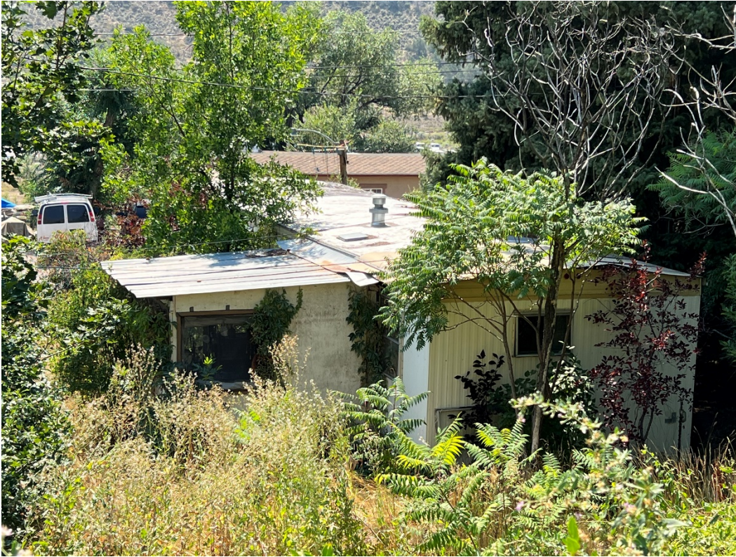
Photo Number: 5GF.5934_1 Description: Looking at the primary (east) and north elevations of the primary trailer. Date: 9/6/2022 View: Southwest
