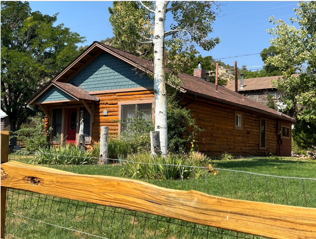
Photo Number: 5GF.5935_2 Description: Looking at the primary (south) and east elevations of the building. Date: 9/6/2022 View: Northwest
