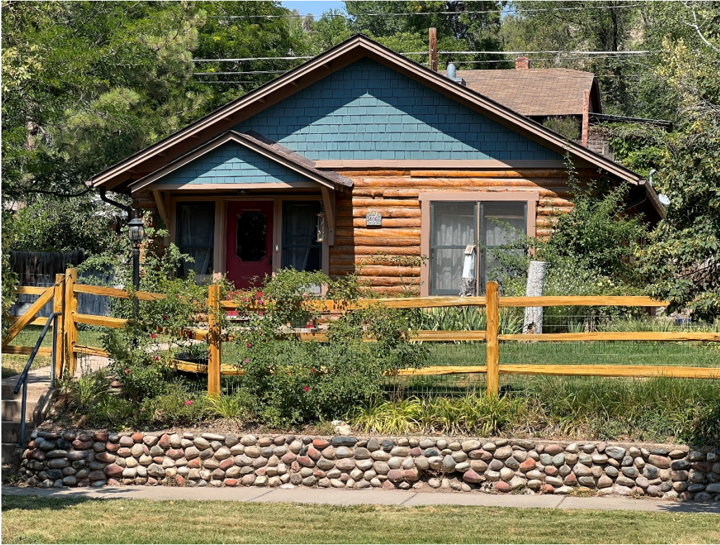
Photo Number: 5GF.5935_1 Description: Looking at the primary (south) elevation of the building. Note the decorative stone masonry wall, and the post and rail fencing. Date: 9/6/2022 View: North
