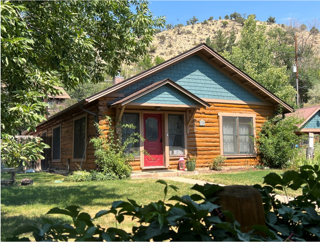
Photo Number: 5GF.5935_3 Description: Looking at the west and primary (south) elevations of the building. Date: 9/6/2022 View: Northeast
