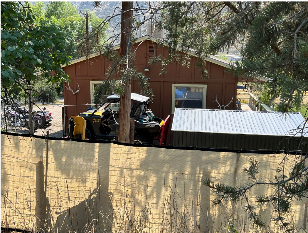
Photo Number: 5GF.5936_2 Description: Looking at the north elevation of the building. Note the horizontal wood belt course in the gable end. Date: 9/6/2022 View: South
