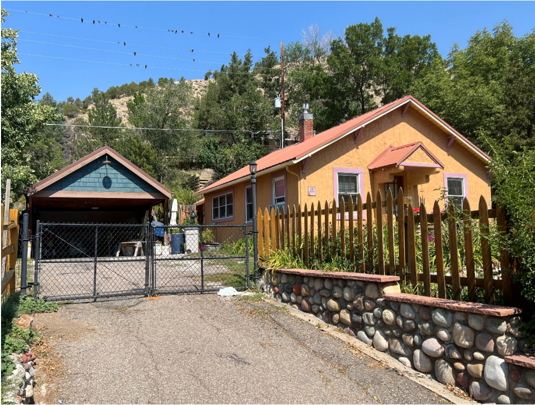
Photo Number: 5GF.5937_3 Description: Context view of the residence's west and primary (south) elevations. Note the stone masonry wall and wood picket fencing along the legal parcel boundary. Date: 9/6/2022 View: Northeast
