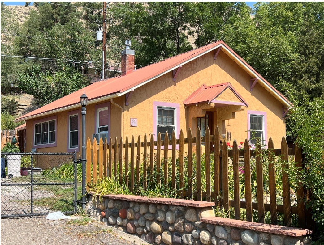
Photo Number: 5GF.5937_2 Description: Looking at the west and primary (south) elevation of the building. Date: 9/6/2022 View: Northeast
