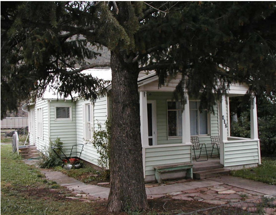
Reference Photo 1 Description: Looking at the east and primary (north) elevation of the building. Date: Circa 2009 View: Southwest
