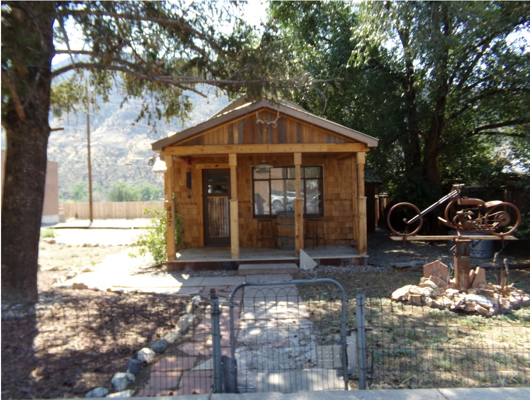
Photo Number: 5GF.5910_1 Description: Looking at the primary (north) elevation of the residence. Date: 9/6/2022 View: South
