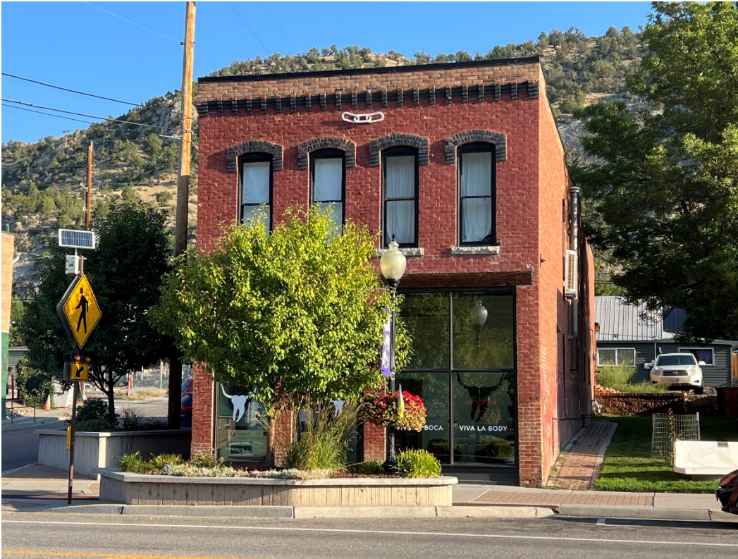
Photo Number: 5GF.1488_1 Description: Looking at the primary (south) elevation of the building. Date: 9/6/2022 View: North
