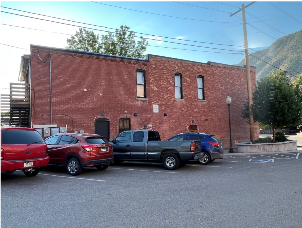
Photo Number: 5GF.1488_4 Description: Looking at the west elevation of the building. Date: 9/6/2022 View: Southeast
