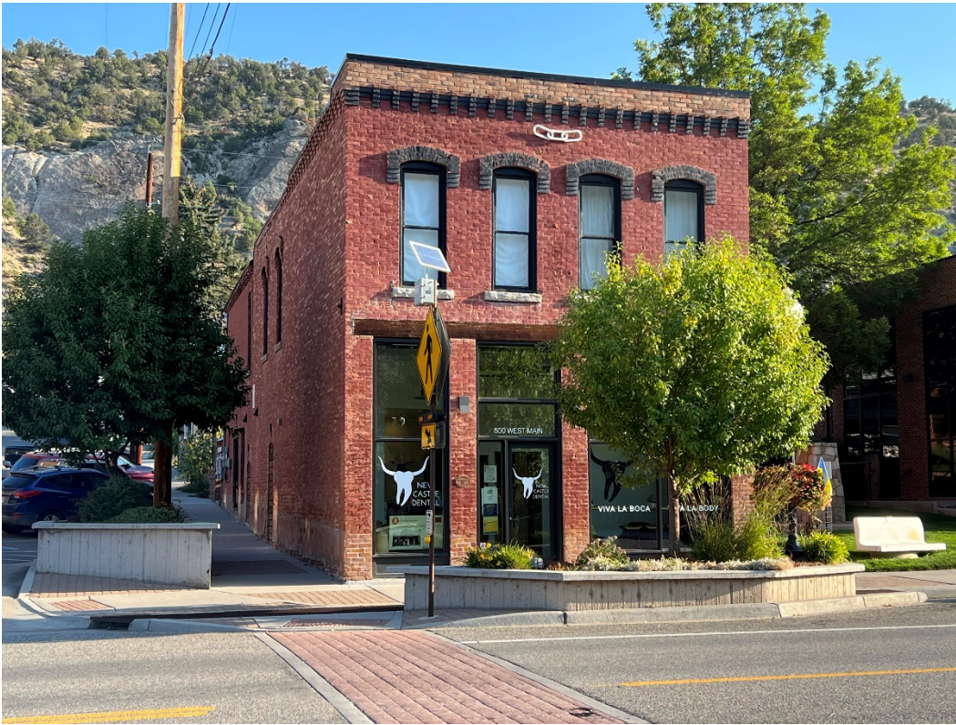
Photo Number: 5GF.1488_3 Description: Looking at the west and primary (south) elevations of the building. Date: 9/6/2022 View: Northeast
