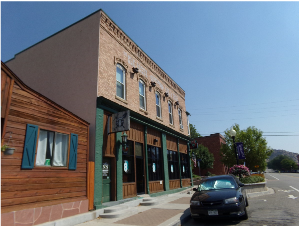
Photo Number: 5GF.1166_1 Description: Looking at the west and primary (south) elevation of the building. Date: 9/6/2023 View: Northeast
