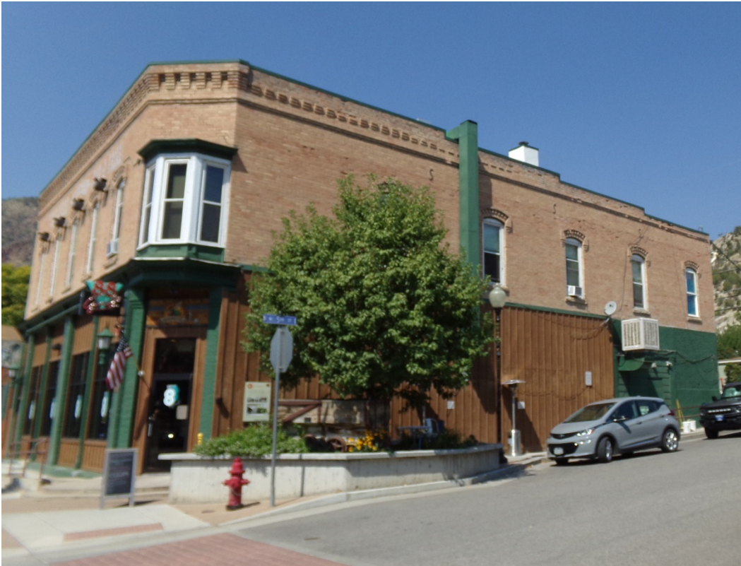
Photo Number: 5GF.1166_1 Description: Looking at the primary (south) and east elevations of the building. Date: 9/6/2022 View: Northwest
