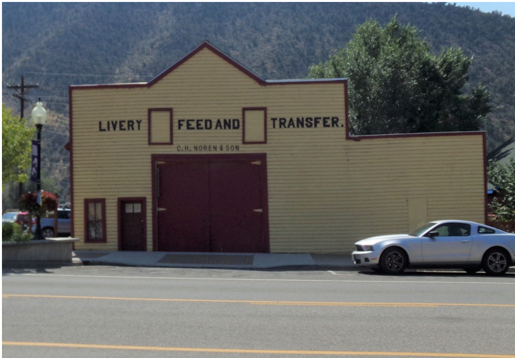
Photo Number: 5GF.2380_1 Description: Looking at the primary (north) elevation of the building. Date: 9/6/2022 View: South
