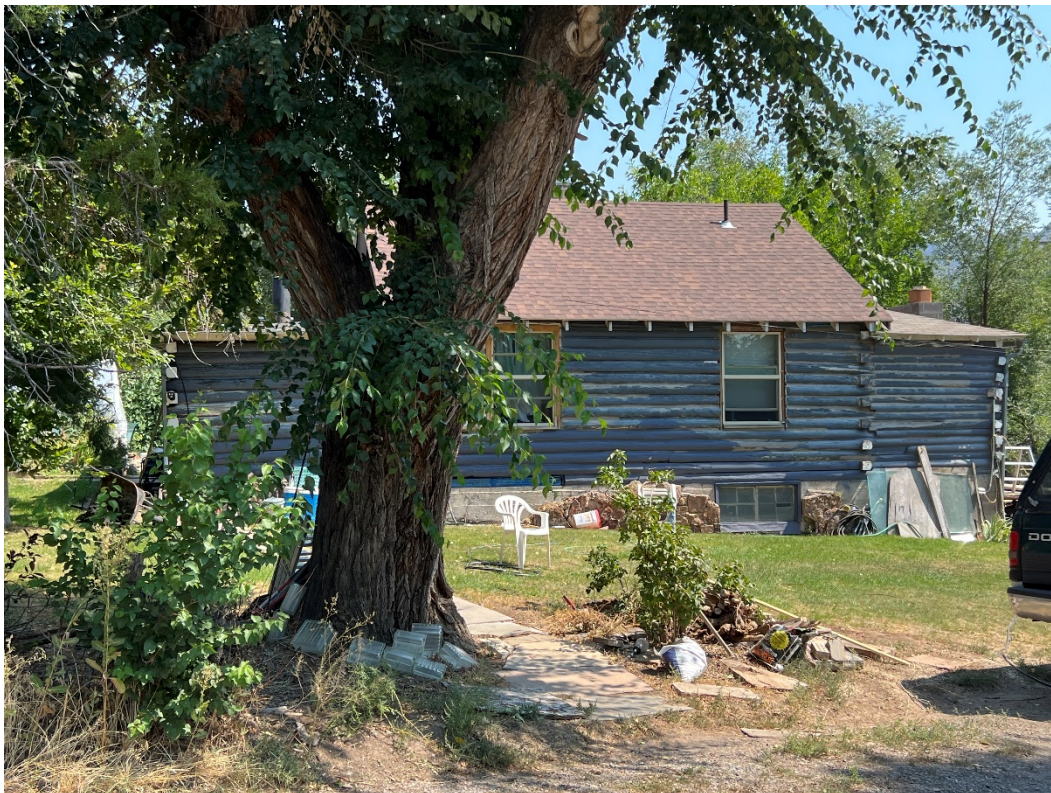
Photo Number: 5GF.5939_4 Description: Looking at the west elevation of the building. Note the CMU block chimney along the south elevation of the building. Date: 9/6/2022 View: East
