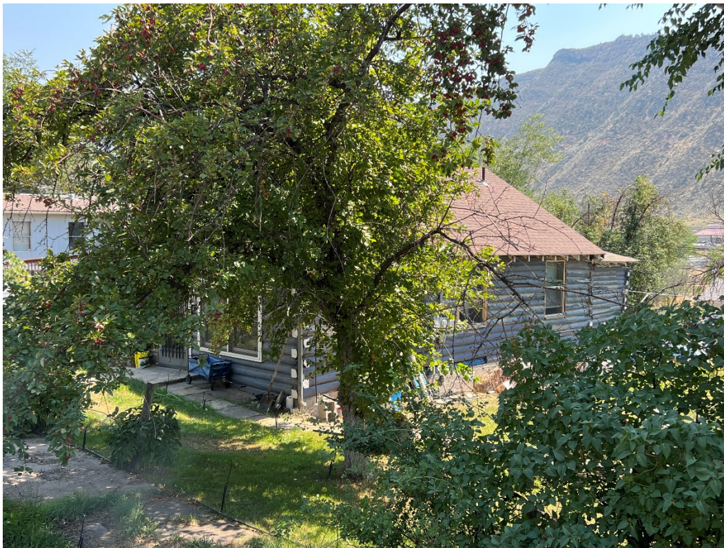
Photo Number: 5GF.5939_3 Description: Looking at an obscured portion of the primary (north) elevation and the west elevation of the building. Date: 9/6/2022 View: Southeast
