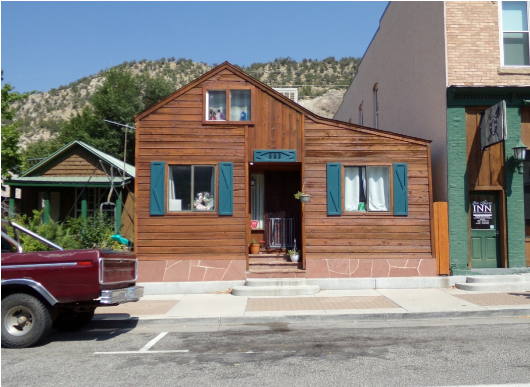
Photo Number: 5GF.5908_1 Description: Looking at the primary (south) elevation. Date: 9/6/2022 View: North
