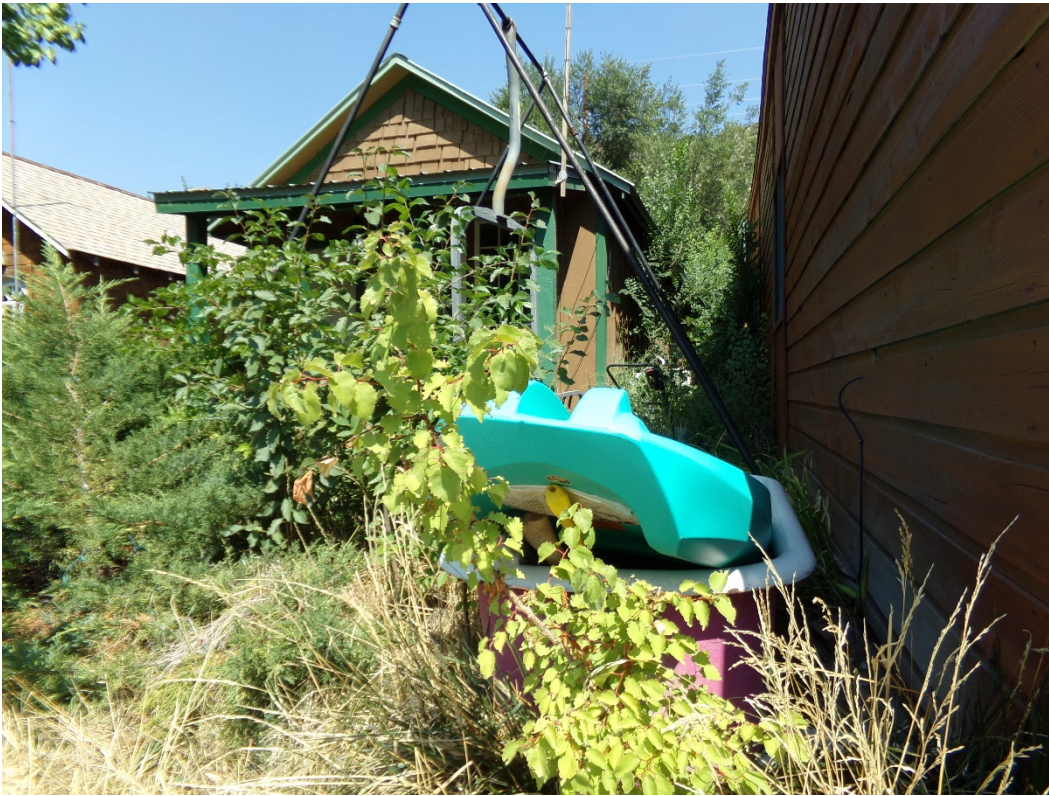
Photo Number: 5GF.5907_3 Description: Looking at the primary (south) and east elevations of the building. Date: 9/6/2022 View: Northwest
