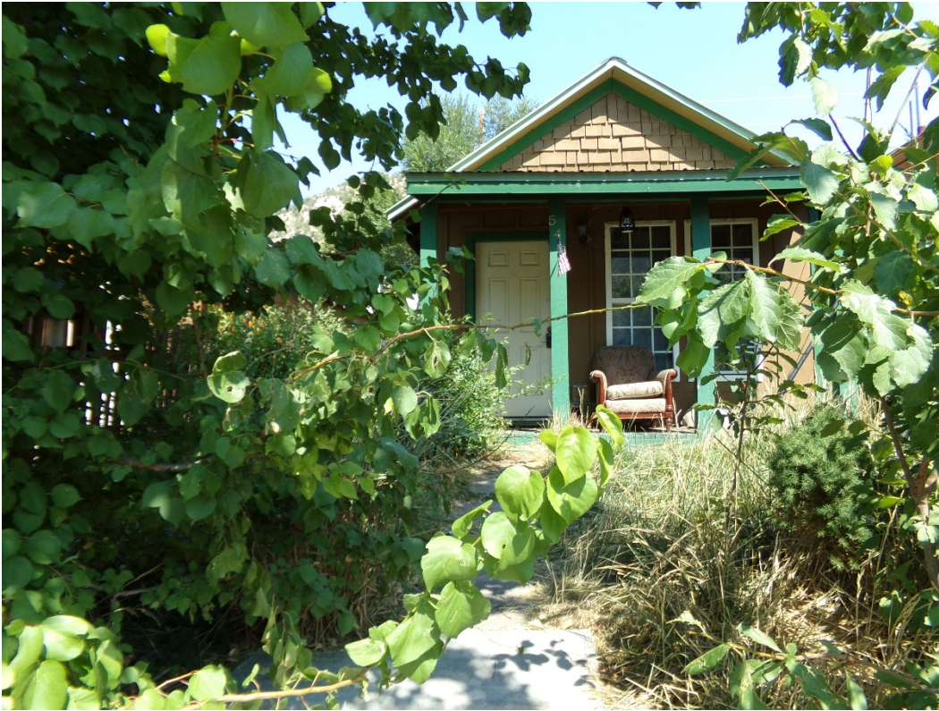
Photo Number: 5GF.5907_1 Description: Looking at the primary (south) elevation of the building. Date: 9/6/2022 View: North
