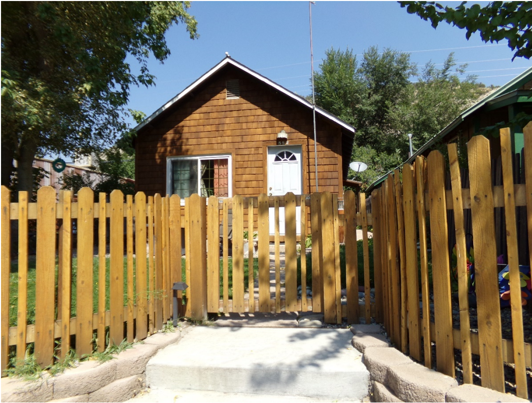
Photo Number: 5GF.5905_1 Description: Looking at the primary (south) elevation of the building. Date: 9/6/2022 View: North
