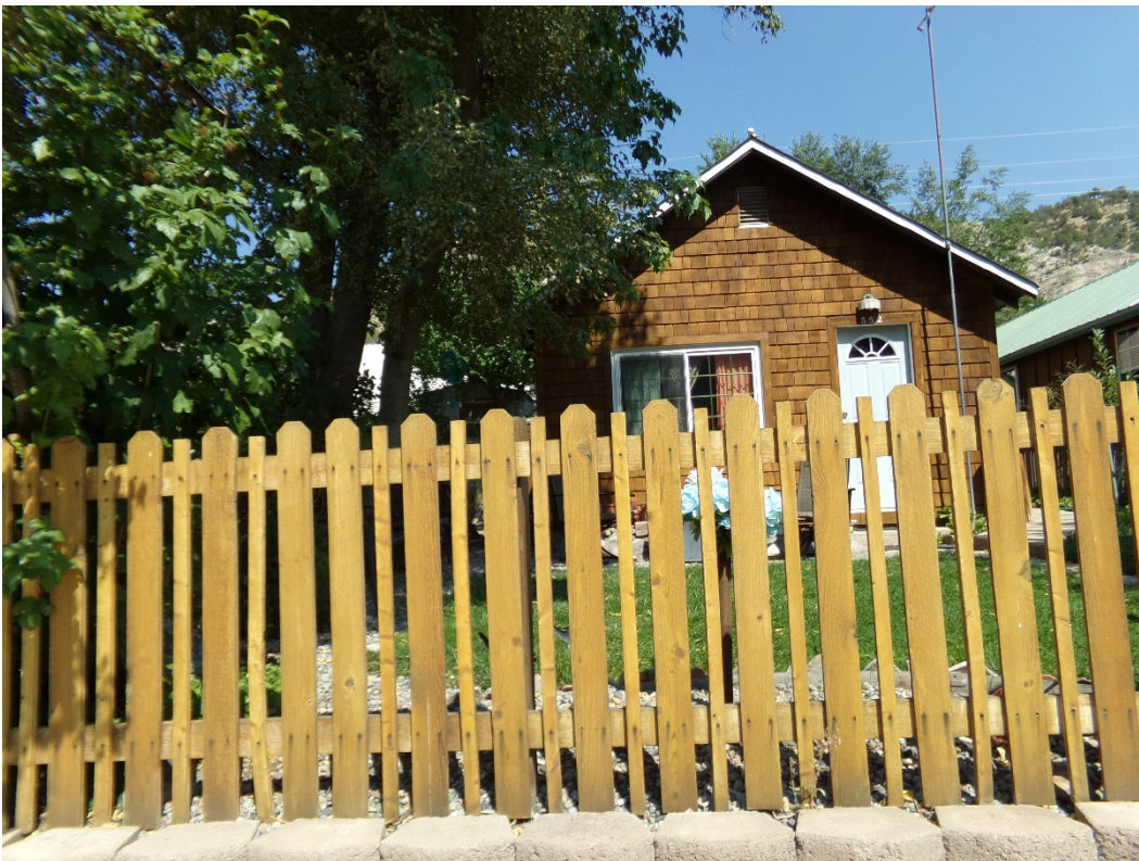
Photo Number: 5GF.5905_2 Description: Looking at the primary (south) elevation of the building. Date: 9/6/2022 View: North
