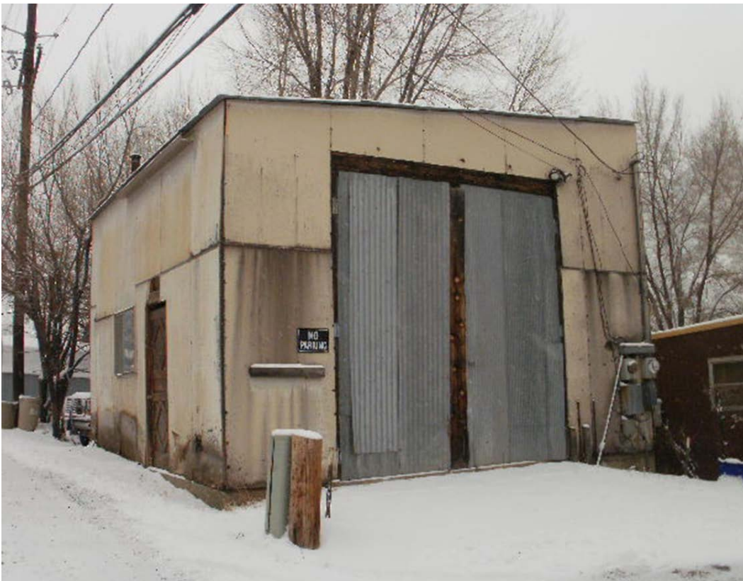
Reference Photo 1 Description: Looking at the north and primary (west) elevation of the outbuilding. Date: circa 2009 Source: Garfield County Assessor's Office
