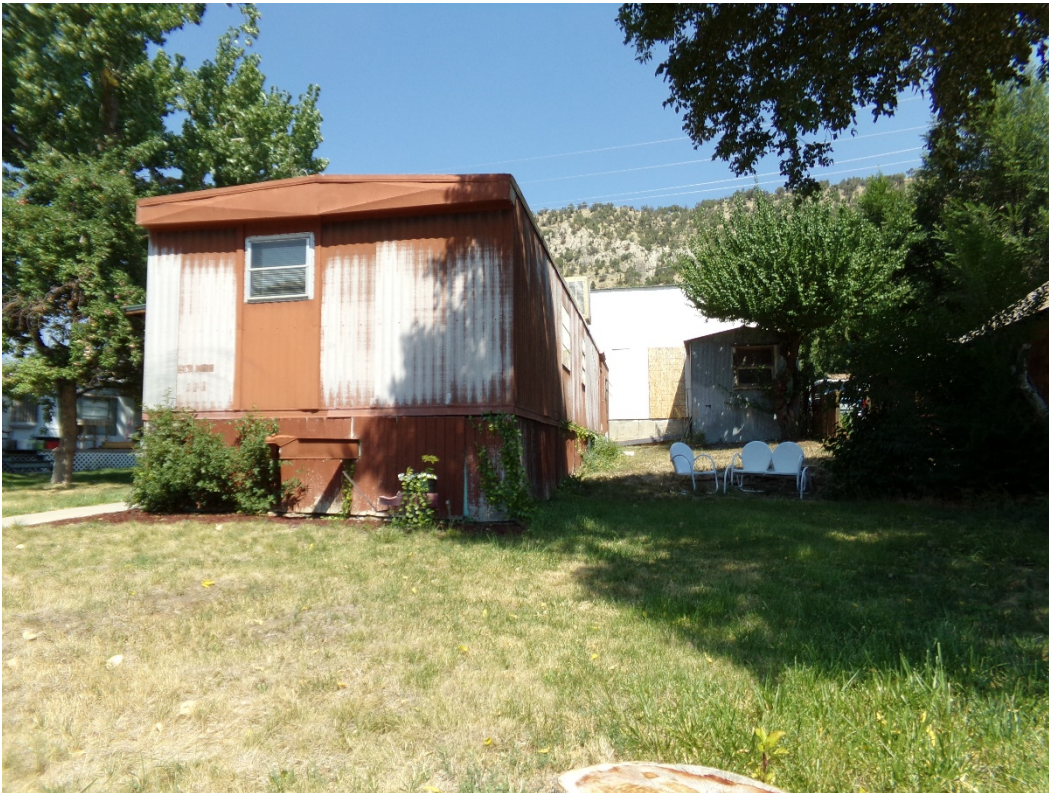
Photo Number: 5GF.5904_3 Description: Looking at the south and east elevations of the trailer. Date: 9/6/2022 View: Northwest
