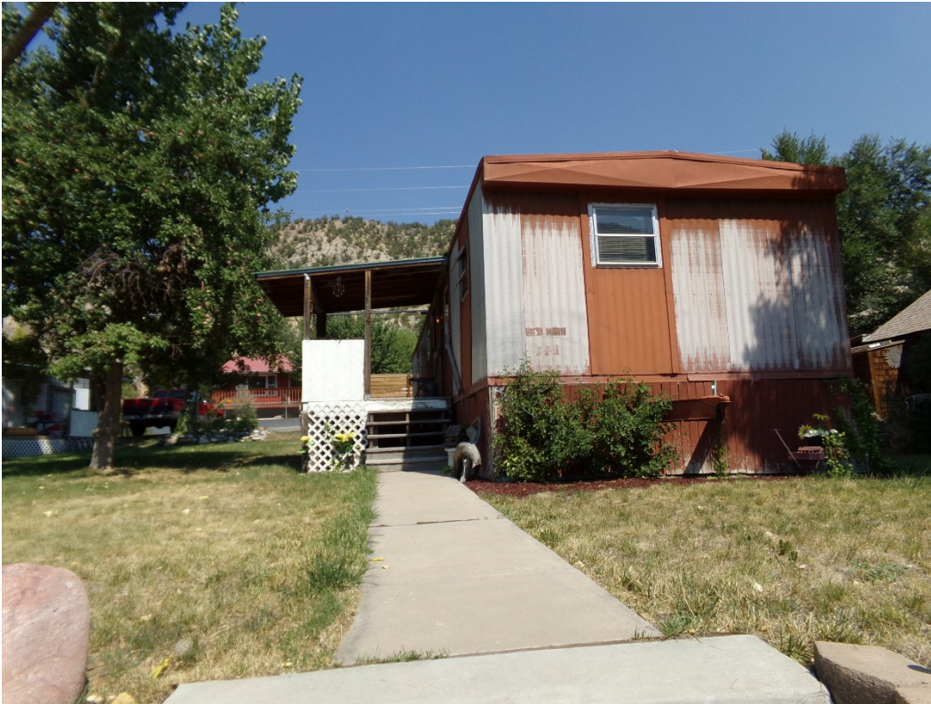
Photo Number: 5GF.5904_1 Description: Looking at the south elevation of the trailer. Date: 9/6/2022 View: North
