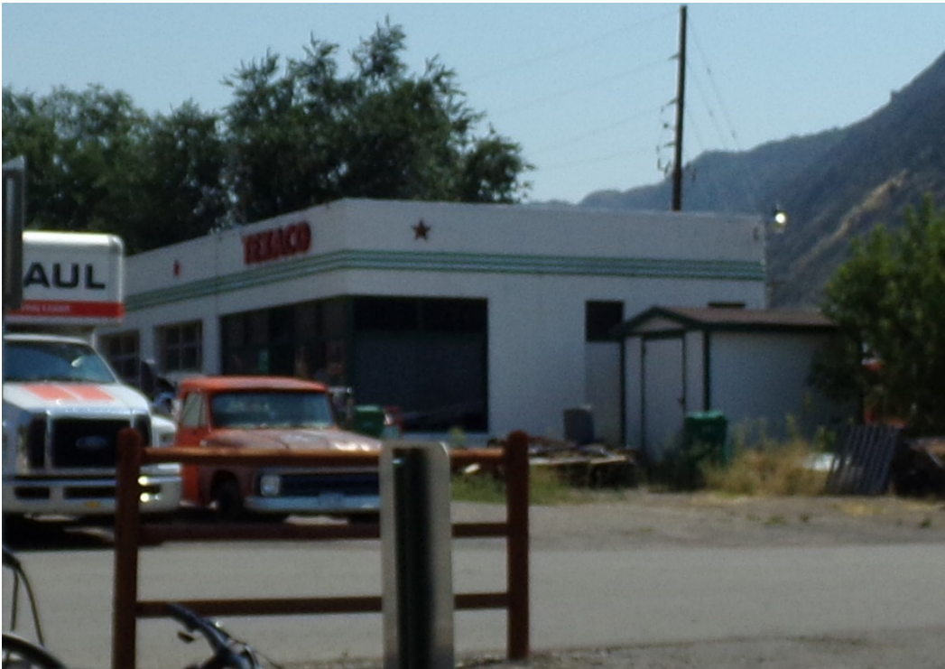
Photo Number: 5GF.5903_3 Description: Looking at the primary (north) elevation and west elevations of the building. Date: 9/6/2022 View: Southeast
