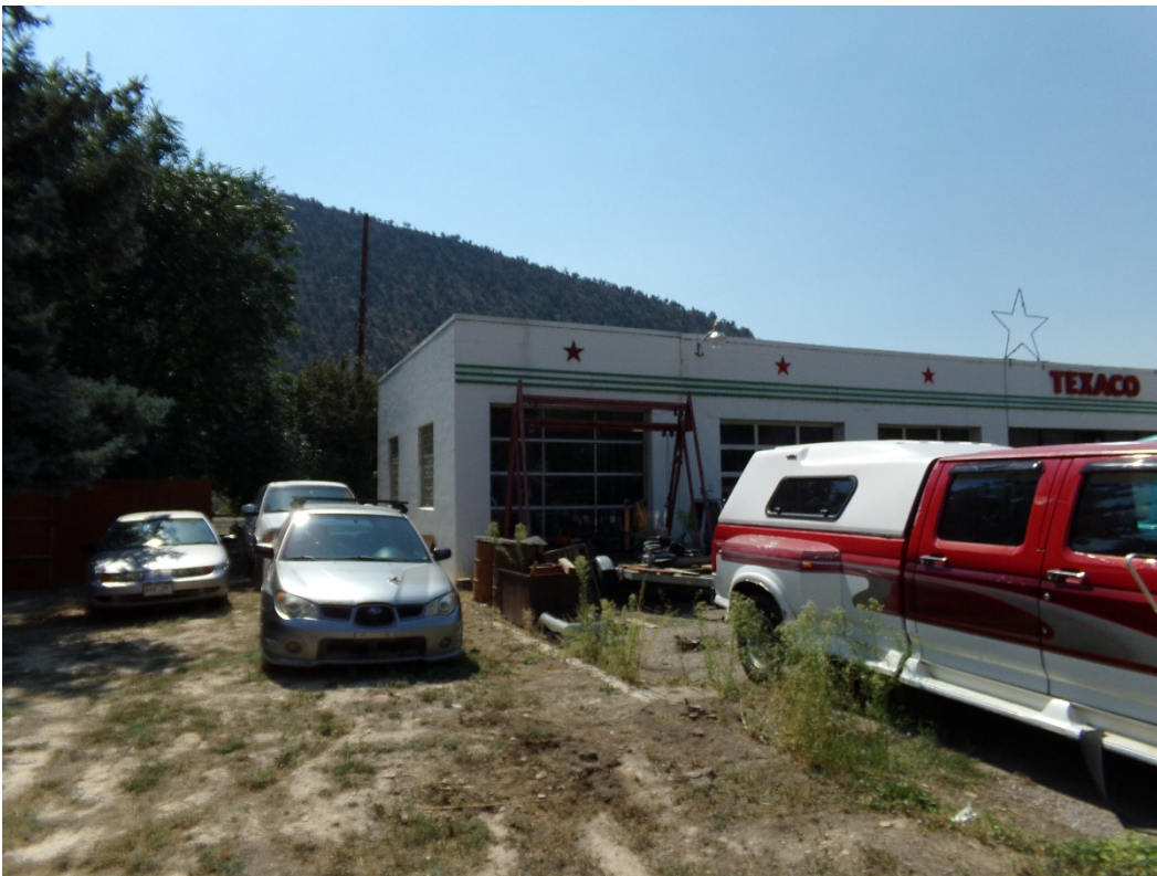
Photo Number: 5GF.5903_4 Description: Looking at the east and primary (north) elevations of the building. The third bay on the far left is likely an addition. Date: 9/6/2022 View: Southwest
