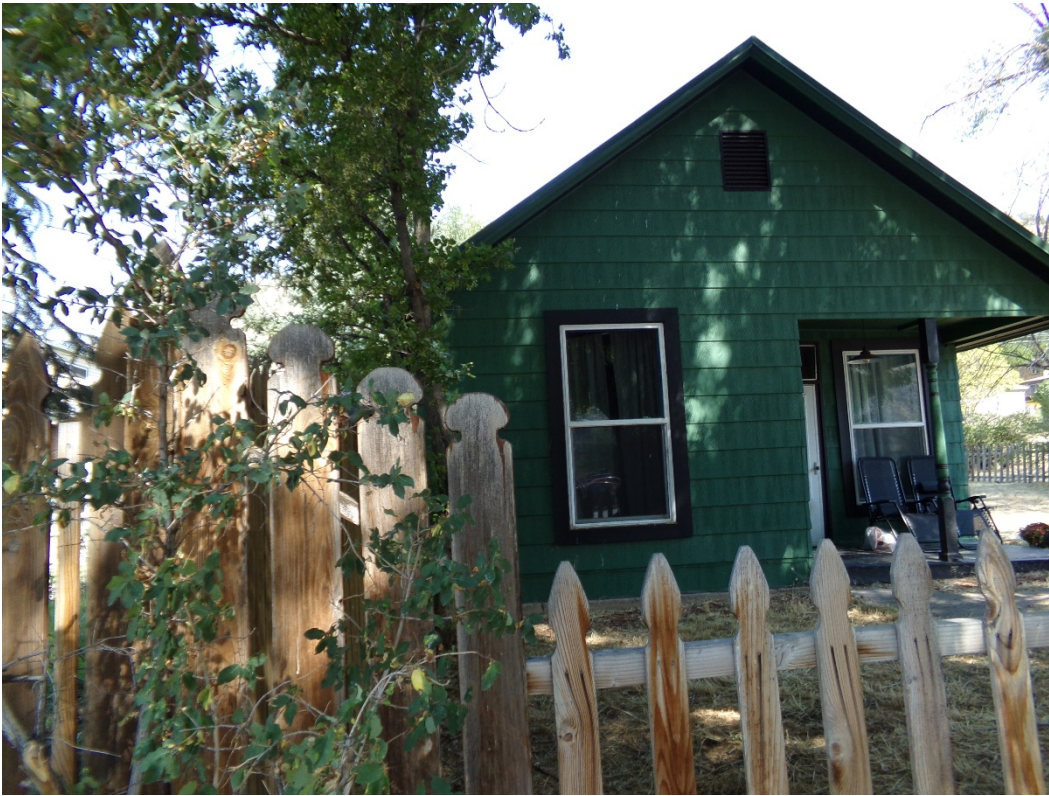
Photo Number: 5GF.5902_3 Description: Looking at the primary (south) elevation of the building. Date: 9/6/2022 View: North
