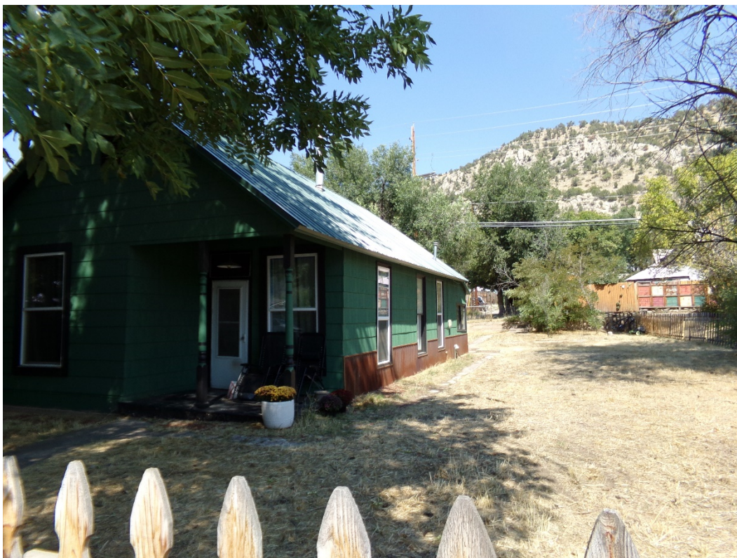
Photo Number: 5GF.5902_2 Description: Looking at the primary (south) and east elevations of the building. Date: 9/6/2022 View: Northwest
