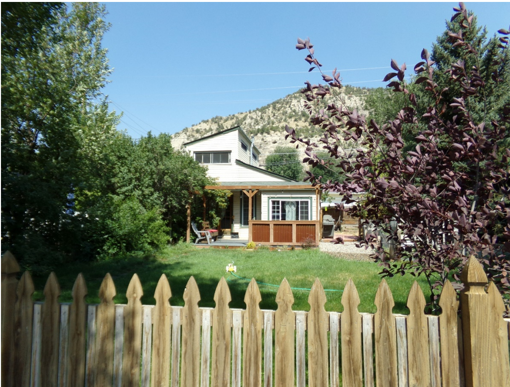
Photo Number: 5GF.5901_1 Description: Context view from Main Street looking at the primary (south) elevation of the building. Date: 9/6/2022 View: North
