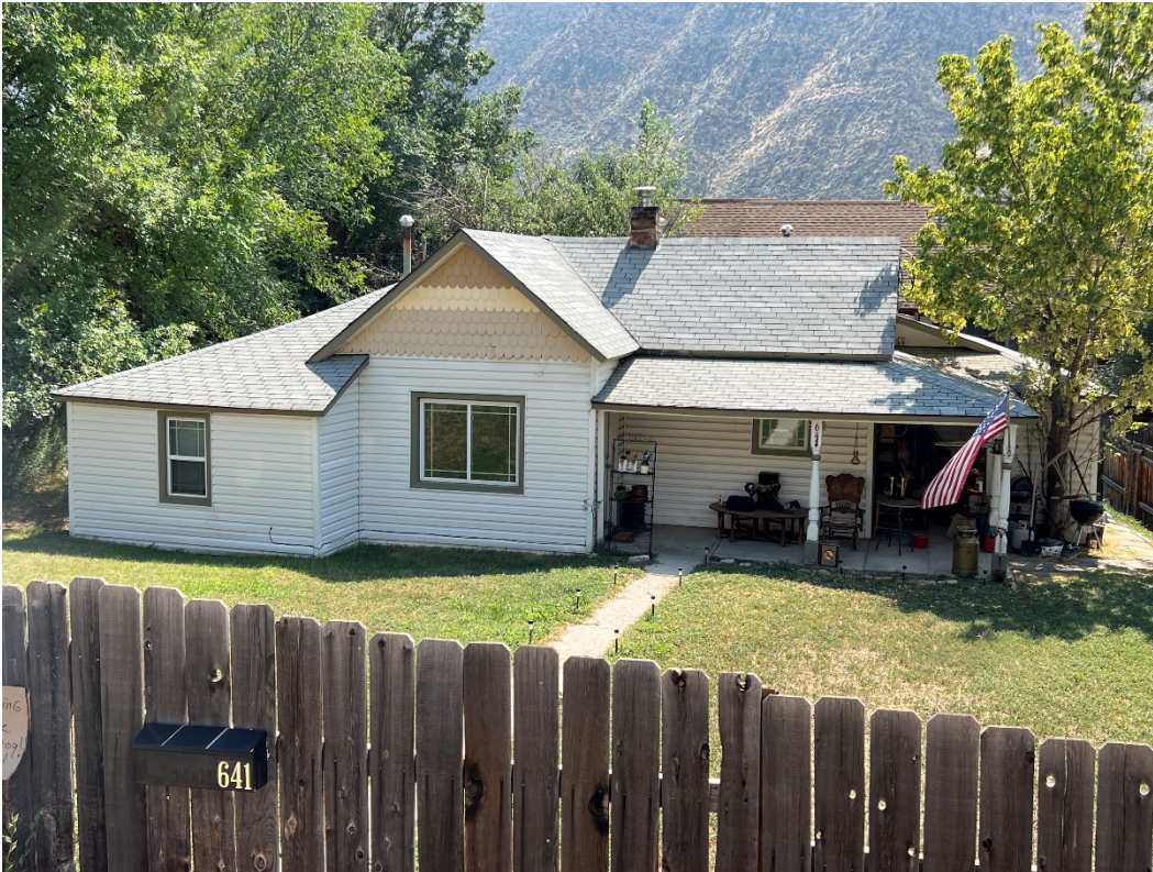
Photo Number: 5GF.5940_1 Description: Looking at the primary (north) elevation of the building. Date: 9/6/2022 View: Southeast
