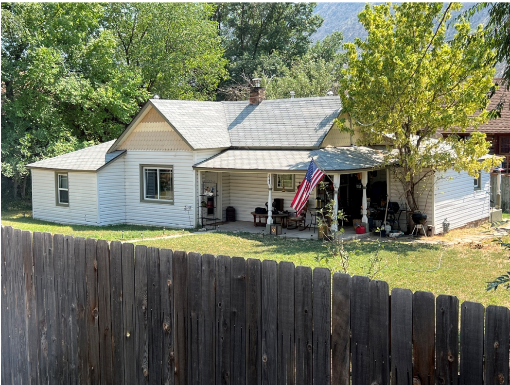
Photo Number: 5GF.5940_2 Description: Looking at the primary (north) and west elevations of the building. Date: 9/6/2022 View: Southeast
