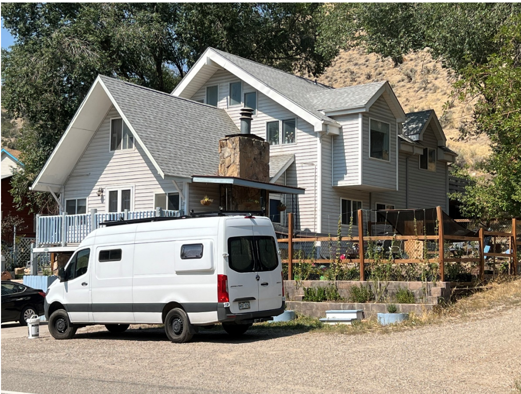
Photo Number: 5GF.5941_2 Description: Looking at the primary (south) and east elevations of the building. Date: 9/6/2022 View: Northwest
