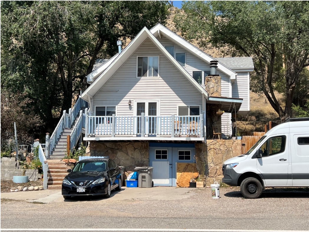
Photo Number: 5GF.5941_1 Description: Looking at the primary (south) elevation of the building. Note the front gable and the side gable projections below the front gable roofline. Date: 9/6/2022 View: North
