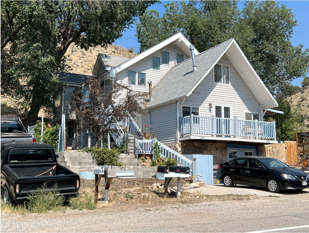
Photo Number: 5GF.5941_3 Description: Looking at the west and primary (south) elevations of the building. Note the staircase leads from the basement level to the second floor. Date: 9/6/2022 View: Northeast
