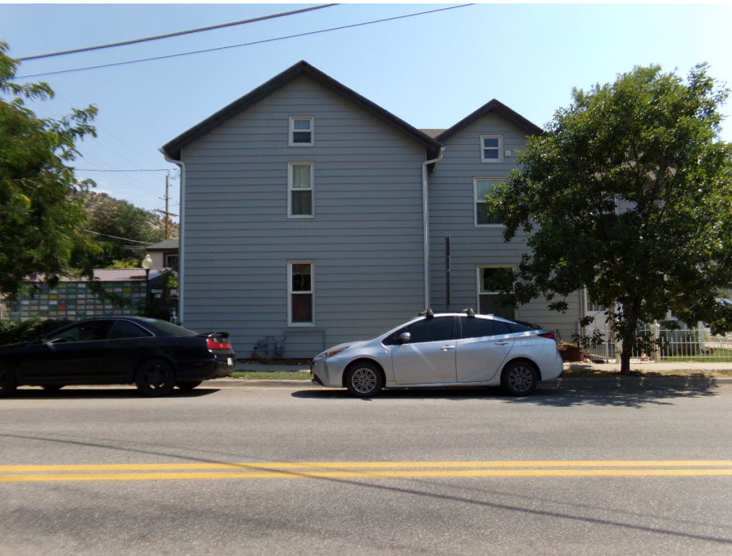
Photo Number: 5GF.5900_4 Description: Looking at the west elevation of the building. Date: 9/6/2022 View: East
