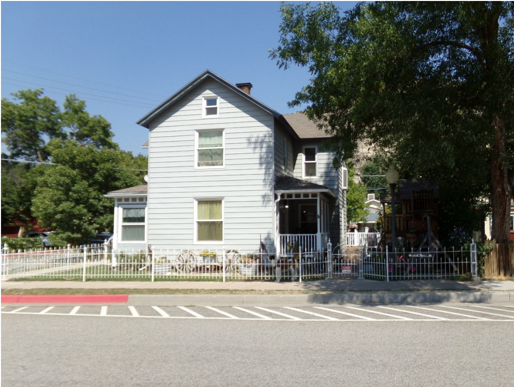
Photo Number: 5GF.5900_1 Description: Looking at the south and primary (east) elevations of the building. Note the decorative wrought iron fence in front of the residence. Date: 9/6/2022 View: Northwest
