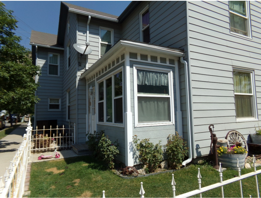
Photo Number: 5GF.5900_3 Description: Looking at the west and south elevations of the building. Date: 9/6/2022 View: Northeast
