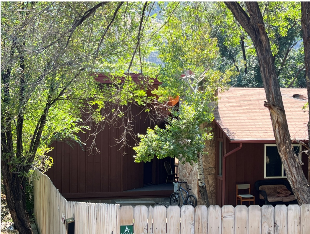
Photo Number: 5GF.5942_2 Description: Close up of the primary (east) elevation of the building. Note the stone masonry chimney. Date: 9/6/2022 View: Southwest
