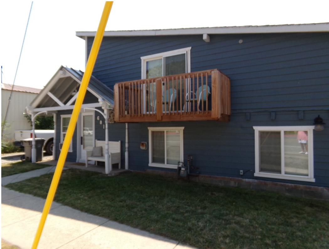
Photo Number: 5GF.5899_1 Description: Looking at the primary (north) elevation of the building. Date: 9/6/2022 View: Southeast
