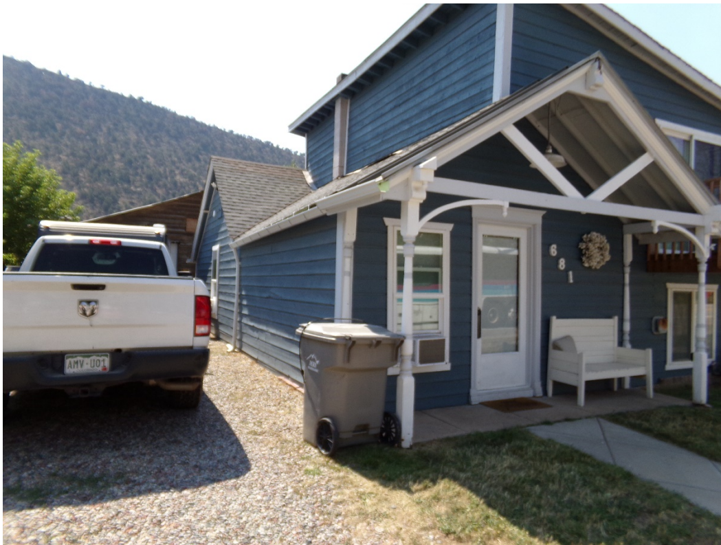
Photo Number: 5GF.5899_2 Description: Looking at the east and primary (north) elevations of the building. Date: 9/6/2022 View: Southwest
