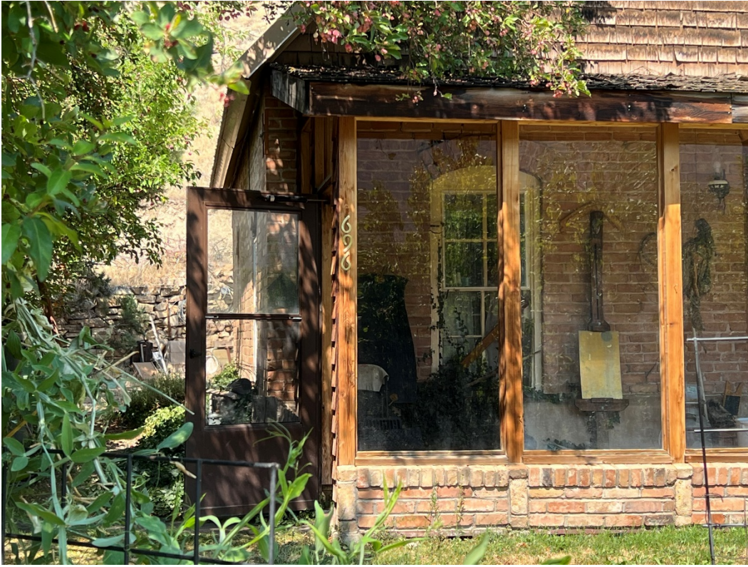
Photo Number: 5GF.5943_3 Description: A small glimpse of the west elevation of the building. Date: 9/6/2022 View: Northeast
