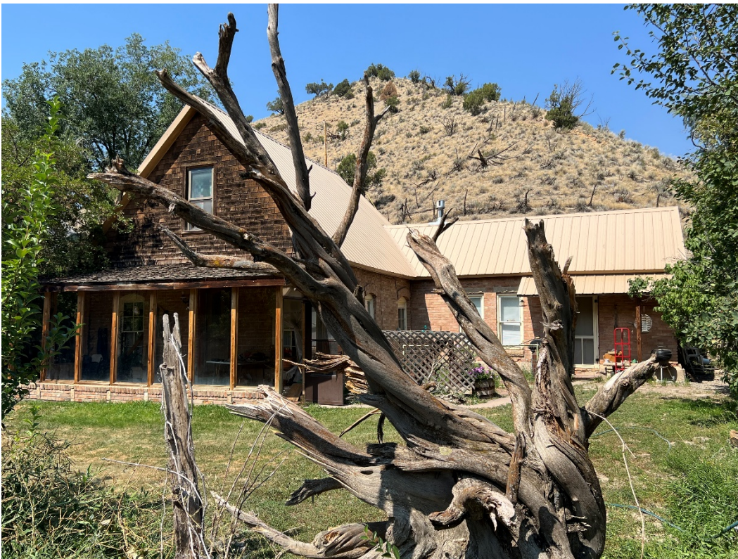
Photo Number: 5GF.5943_2 Description: Looking at the entire facade of the primary (south) elevation. Note the wood shingle exterior in the gable end while brick masonry cladding encompasses the right side of the building. Date: 9/6/2022 View: Northwest
