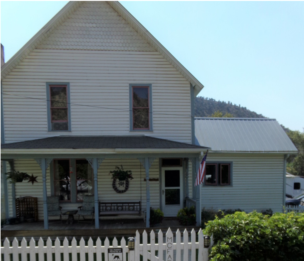
Photo Number: 5GF.5897_3 Description: Looking at the primary (north) elevation of the building. Date: 9/6/2022 View: South
