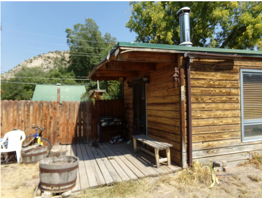
Photo Number: 5GF.5896_2 Description: Looking at the right side of the primary (west) elevation of the building. View: Northeast
