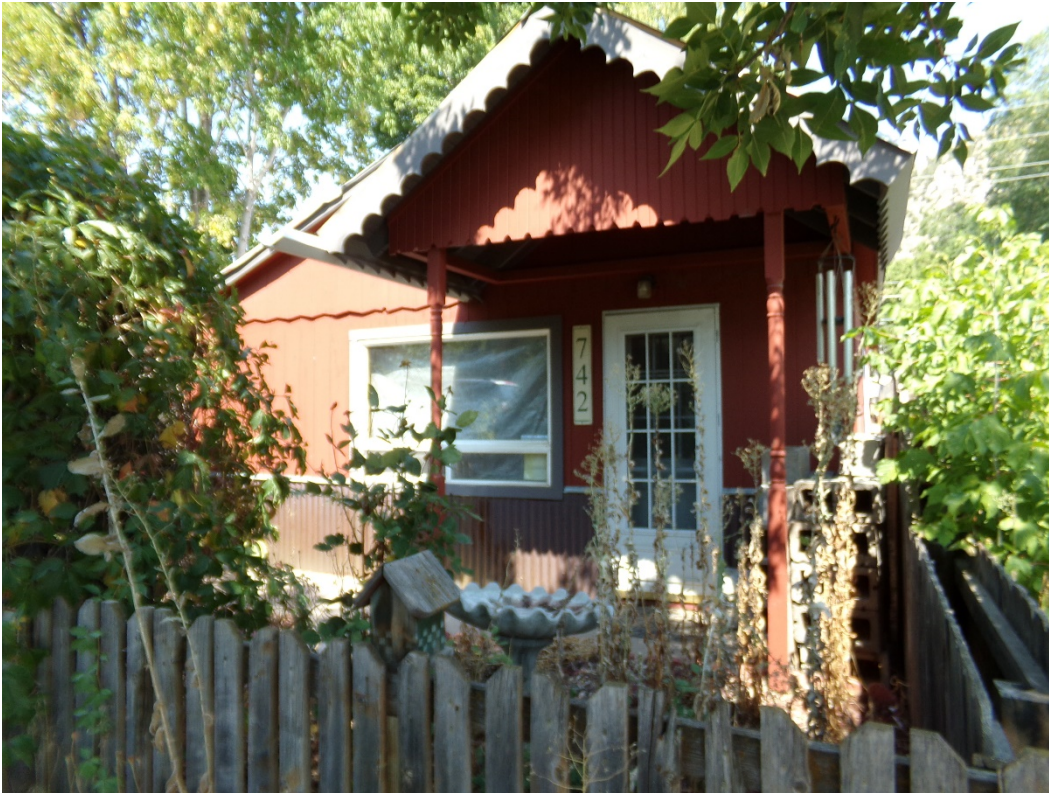
Photo Number: 5GF.5895_1 Description: Looking at the primary (south) elevation of the building. Date: 9/6/2022 View: Northwest
